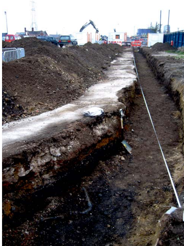
Fig 3a Photograph showing the excavation of the cable trench
