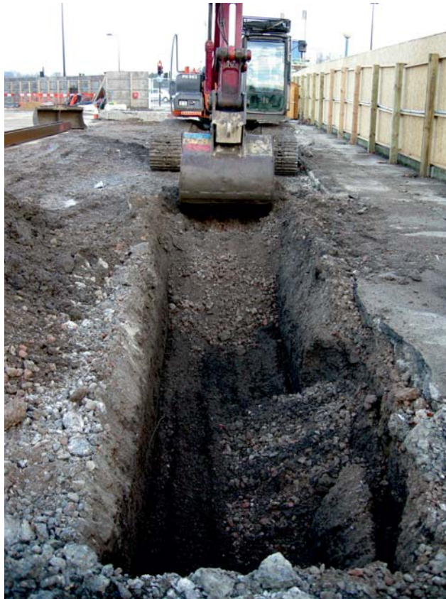
Fig 4 Photograph showing the excavation within the 'strip map and sample' area
