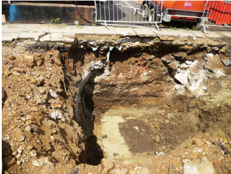
Photo 3: Trench 2, looking east (west-facing section and base of trench) showing Albion Brewery Concrete foundations cutting through archaeologically sterile natural deposits
