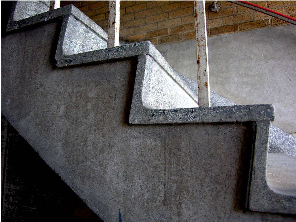
Fig 22 The terrazzo covered steps of Area 3, looking south
