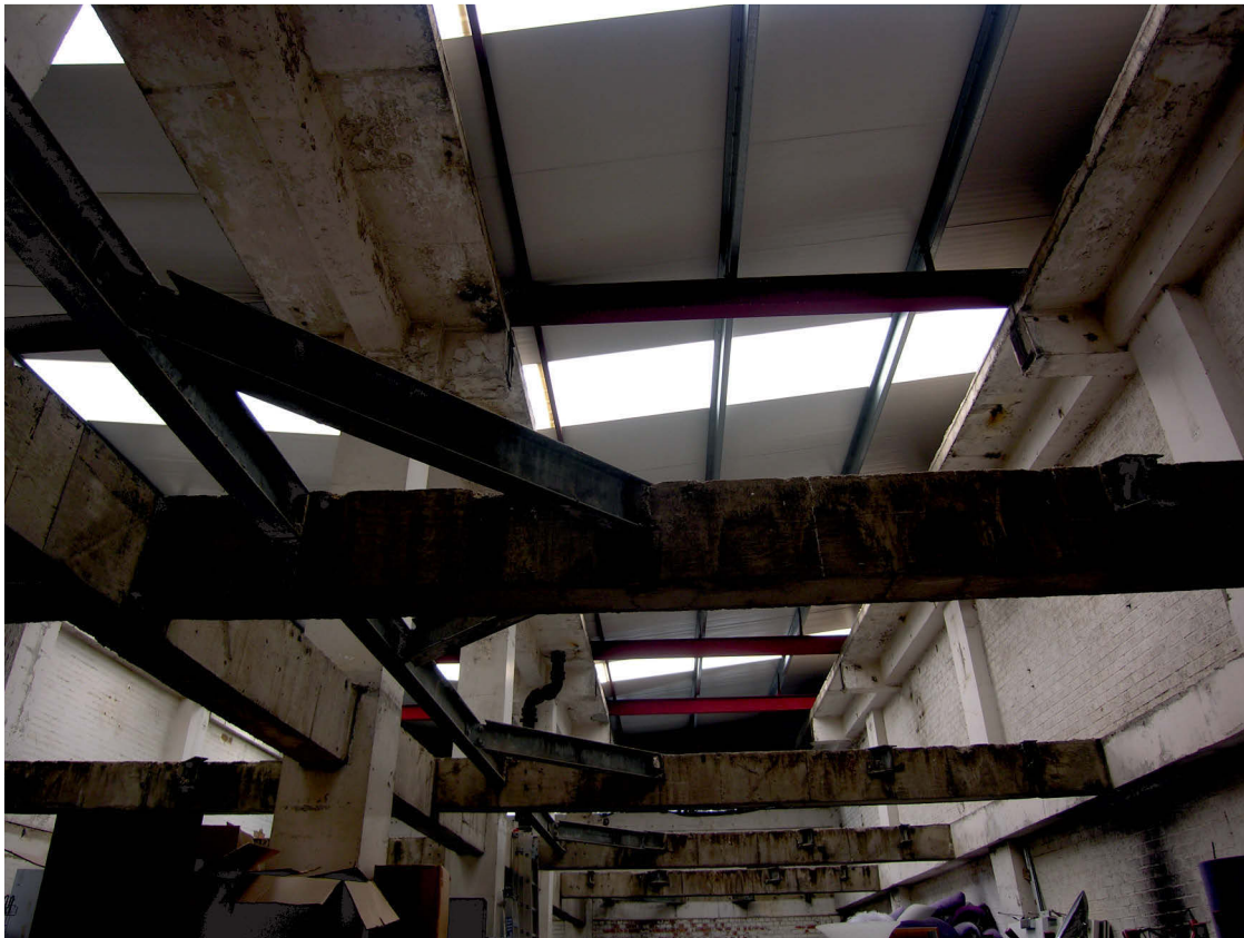
Fig 18 The vat housing structure within Area 2, looking south
