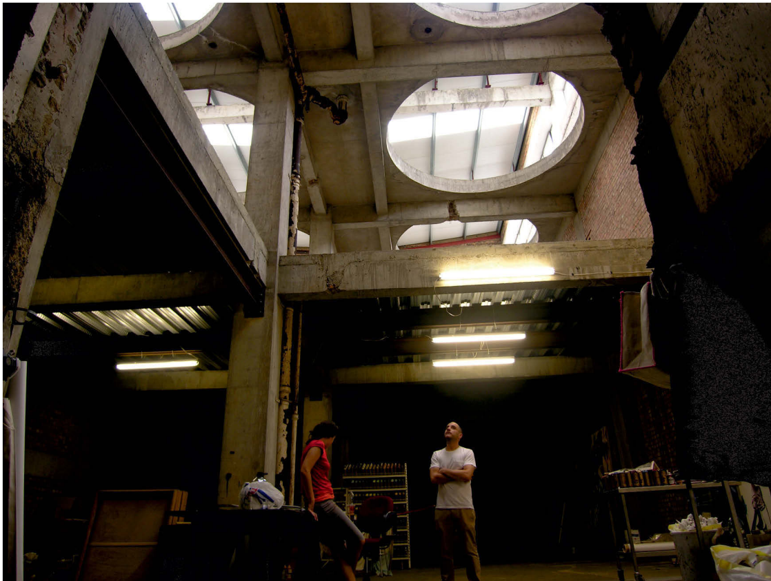
Fig 12 The recently inserted 1st floor of Area 1, looking south
