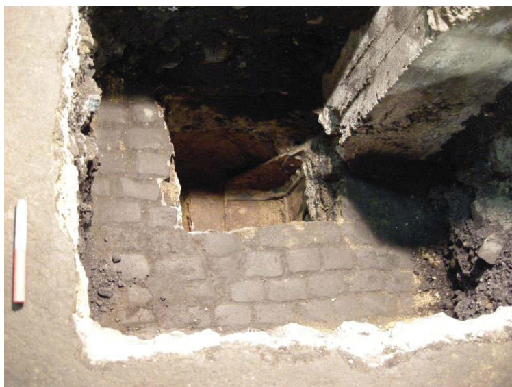
Fig 3 Column base in TP544
