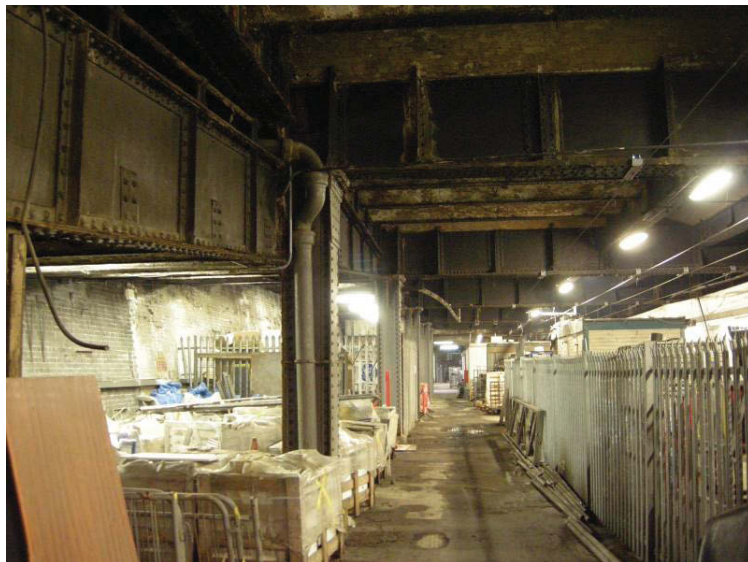
Fig 4 Back of houses showing columns and brick wall
