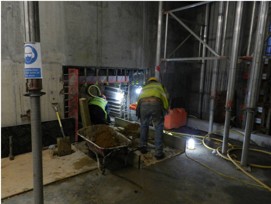
Fig 3 The sewer heading
