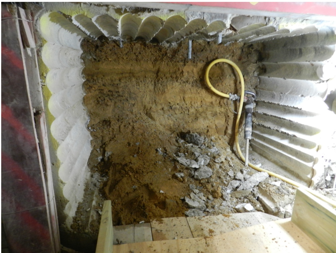
Fig Natural sand and gravels in the sewer heading
