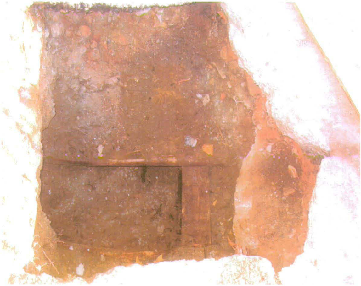
Fig 3 Trial Hole A looking east
