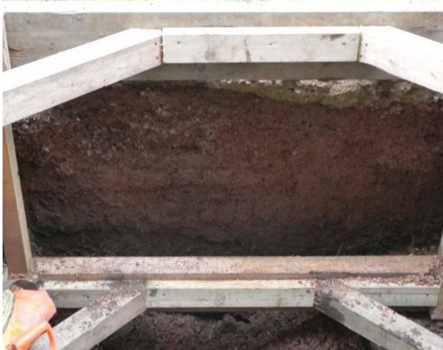
Photo 4: Trench 14 – c 19th-century arched brick foundation beyond the southern limit of the trench, looking south.
