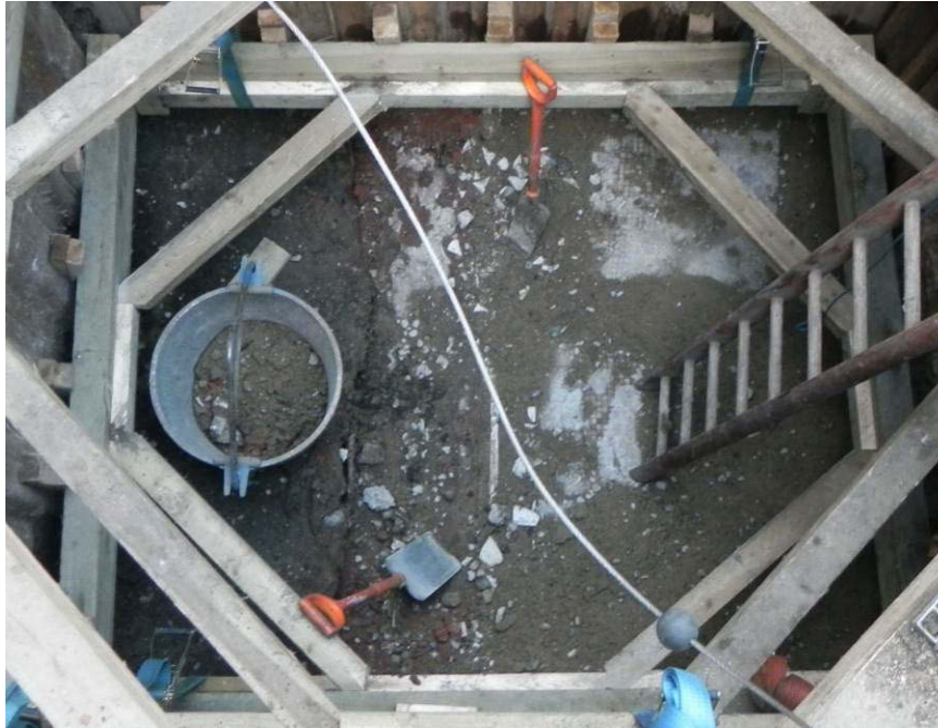
Photo 7: Pit 1 - 20th-century subterranean public toilet block [887], wall left and the surface of tiled floor right, at 109.09m ATD (3.20m bGL) being broken out, west at top.
