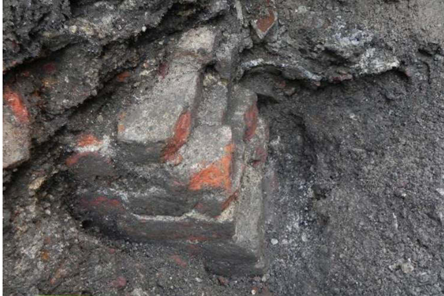
Photo 22: Brick wall [915] in SSET/UKPN Diversion Trench, truncated on the right by utilities, looking west.
