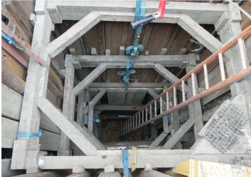
Photo 18: Pit 10 – Excavated into natural gravel [924], showing the base of the pit at 107.21m ATD (5.70m bGL), south at top.
