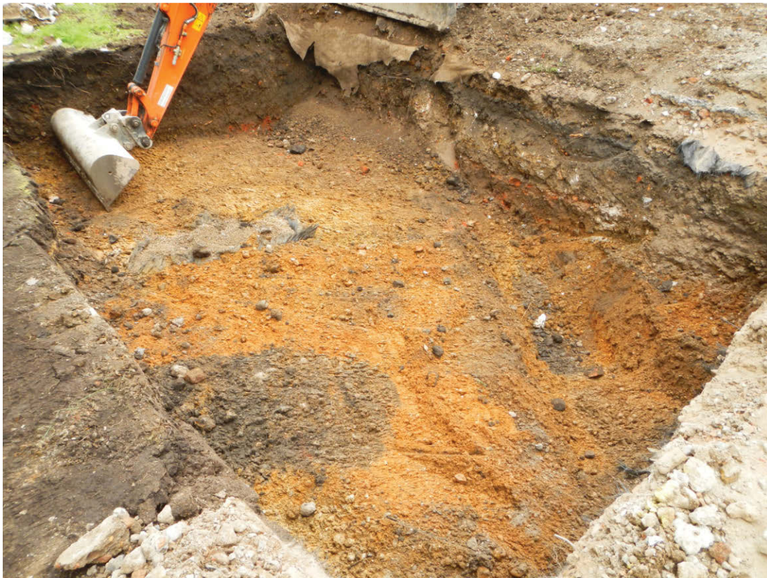
Fig 6 Eastern soakaway being excavated, looking north
