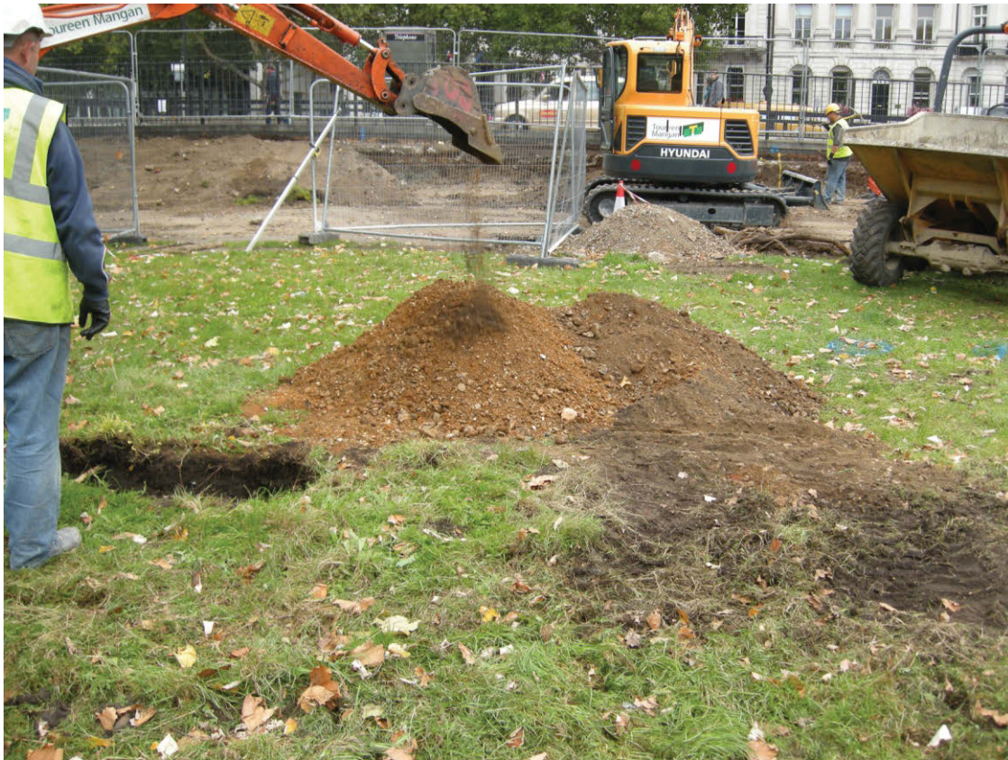
Fig 5 Example of pile probing, looking north
