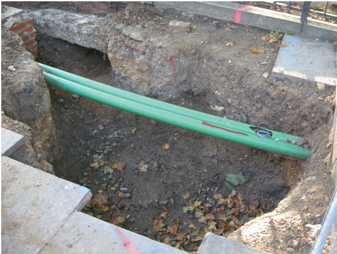
Fig 4 Diversion of services looking north
