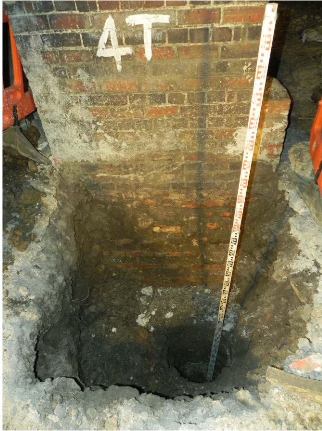
Photo 10 19th-century brick offsets and column, looking west.
