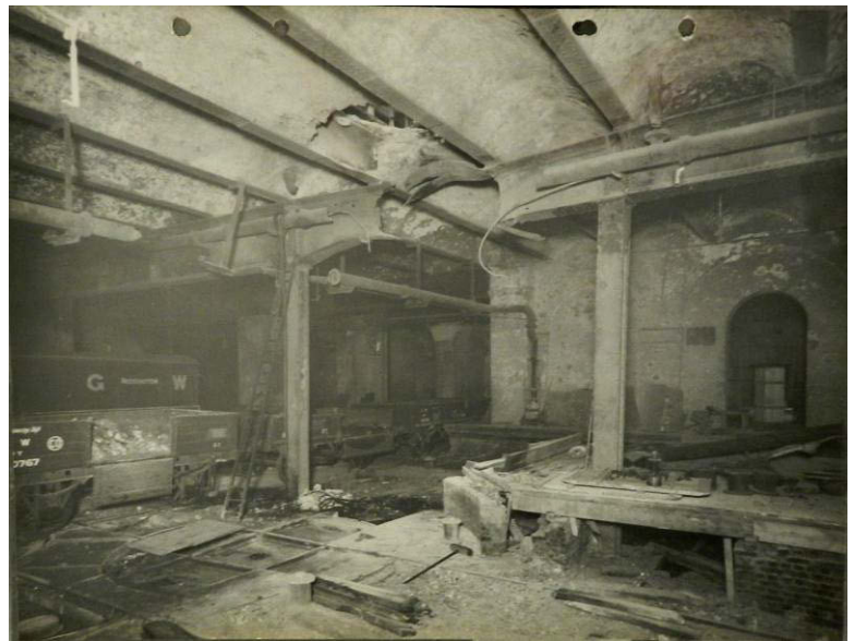
Photo 19 Photograph of the terminus following the WWII explosion, 1940, showing one of the platforms. Note the brick supporting wall clearly shown in the bottom right hand corner (COL/AC/23/0122)
