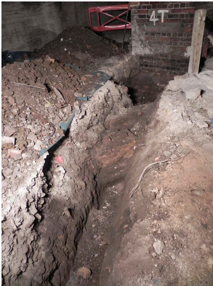
Photo 13, two parallel walls [86] and [88], possibly denoting the northern edge of a '19th-century] platform, looking south-east.
