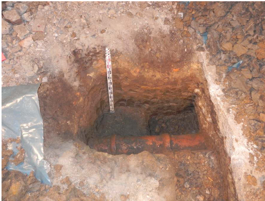
Photo 12, 19th-century drain overlain by 20th-century concrete foundation (right of picture), looking south.
