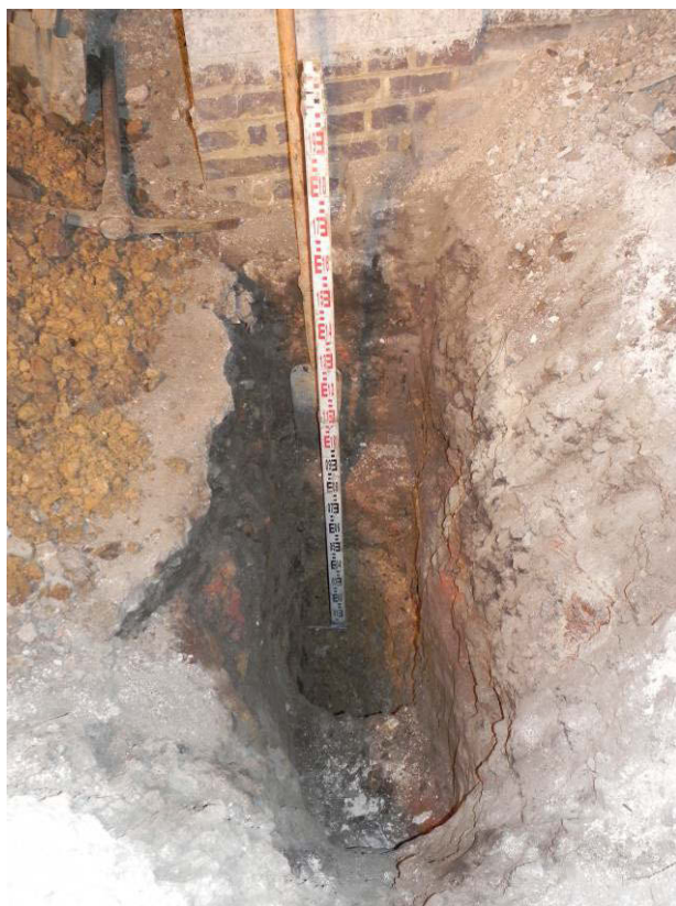
Photo 9, 20th-century foundations abutting earlier structures, looking north.
