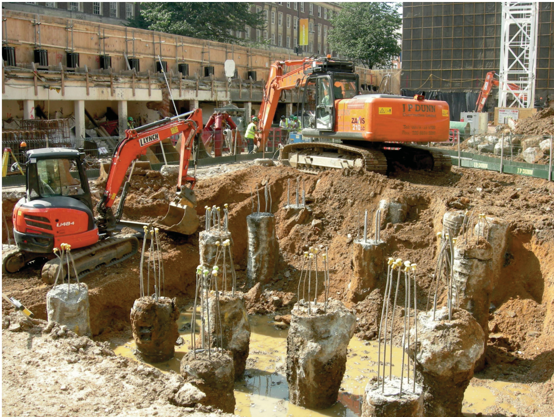
Fig 3 Photograph showing ground reduction on south side of site (looking NW)
