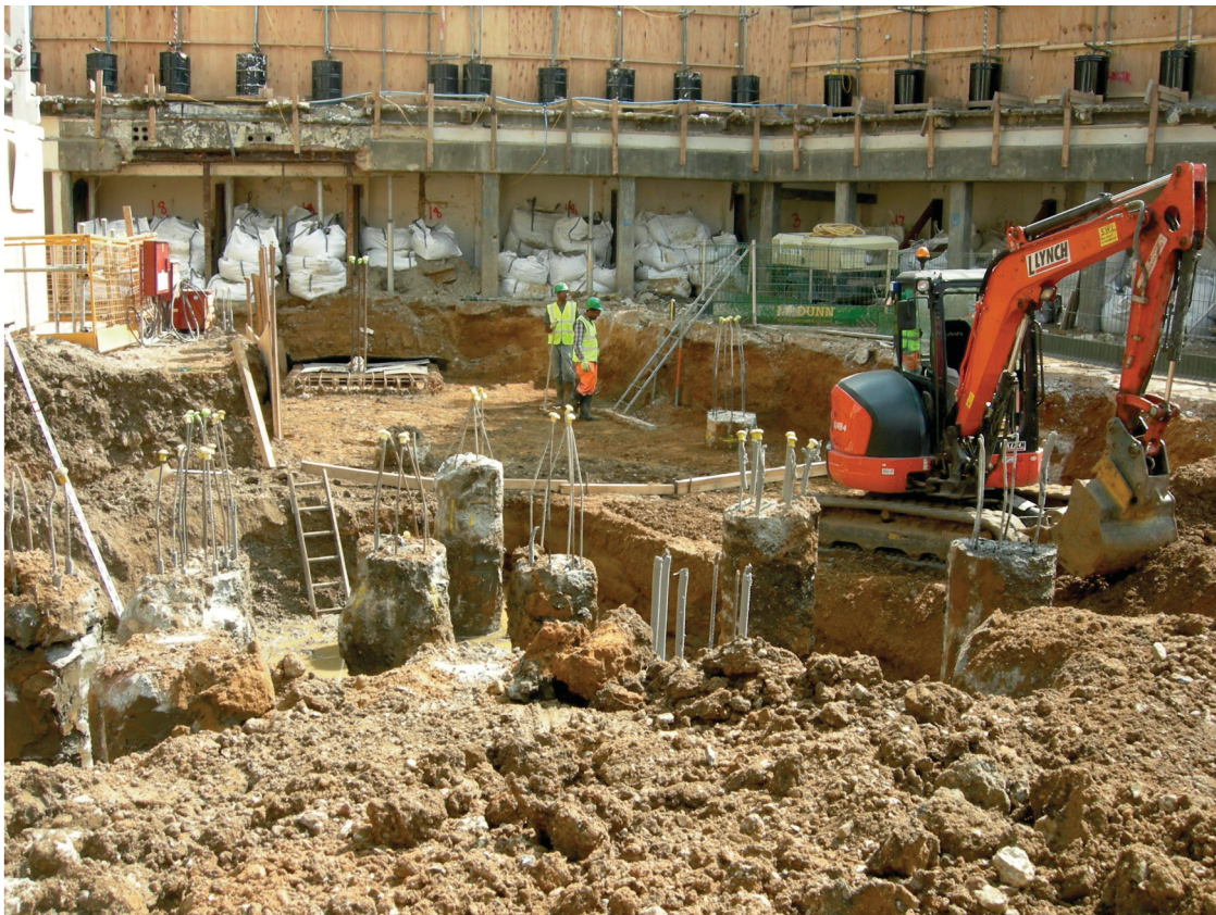
Fig 4 Photograph showing ground reduction on south side of site (looking SE)
