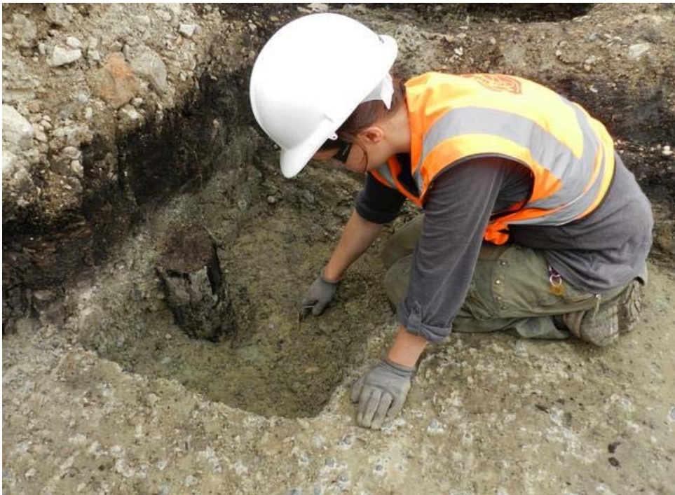
Photo 3 Trench 1B: Excavating timber [11] in the southeast corner (looking southwest)
