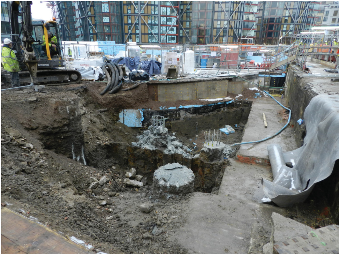
Fig 3 Crane base trench (looking west)
