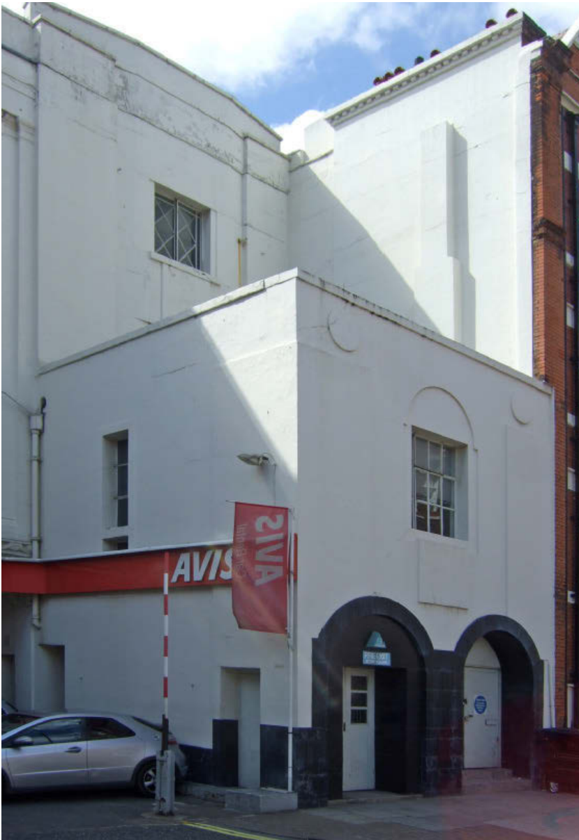
Fig 20 Exterior of the garage on Balderton Street and the east opening to the ground-level passage to St Mark's Church, looking south-west (Heyne Tillett Steel 2009)
