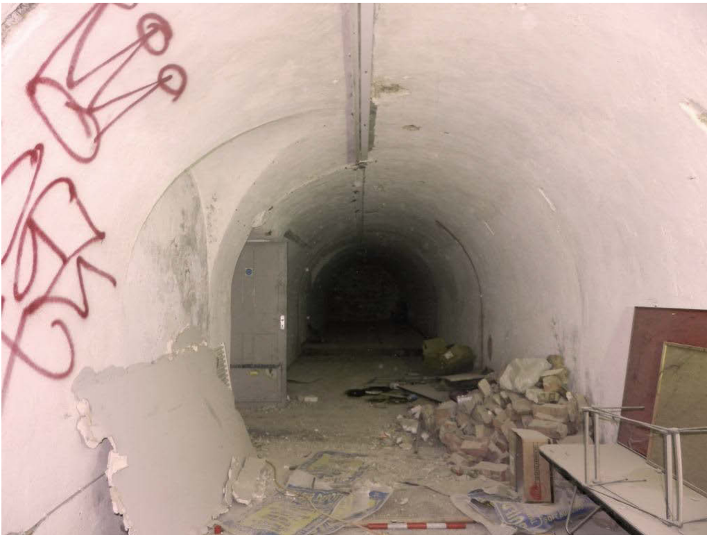
Fig 17 The northern vault looking west, showing an opening on the south groined into the vault, later blocked, and the entrance of 1925-26 (MOLA image 35)
