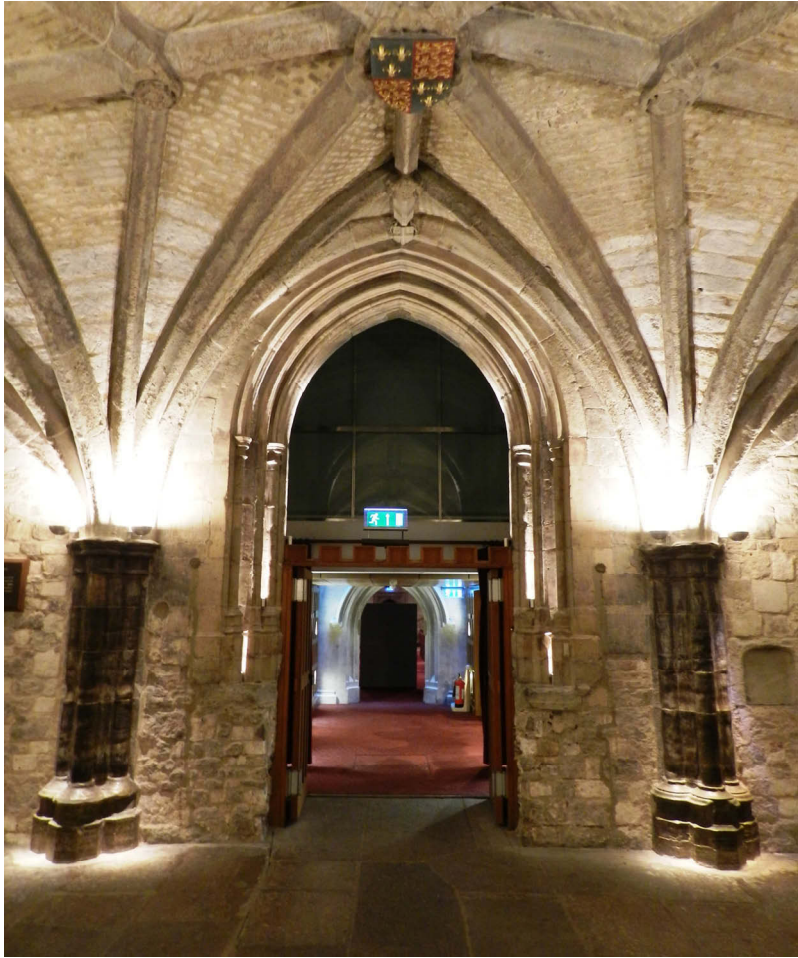
Fig 3 The east door of the East Crypt, looking east. Note the difference in height between the ground level and the base of the orders of pilasters.
