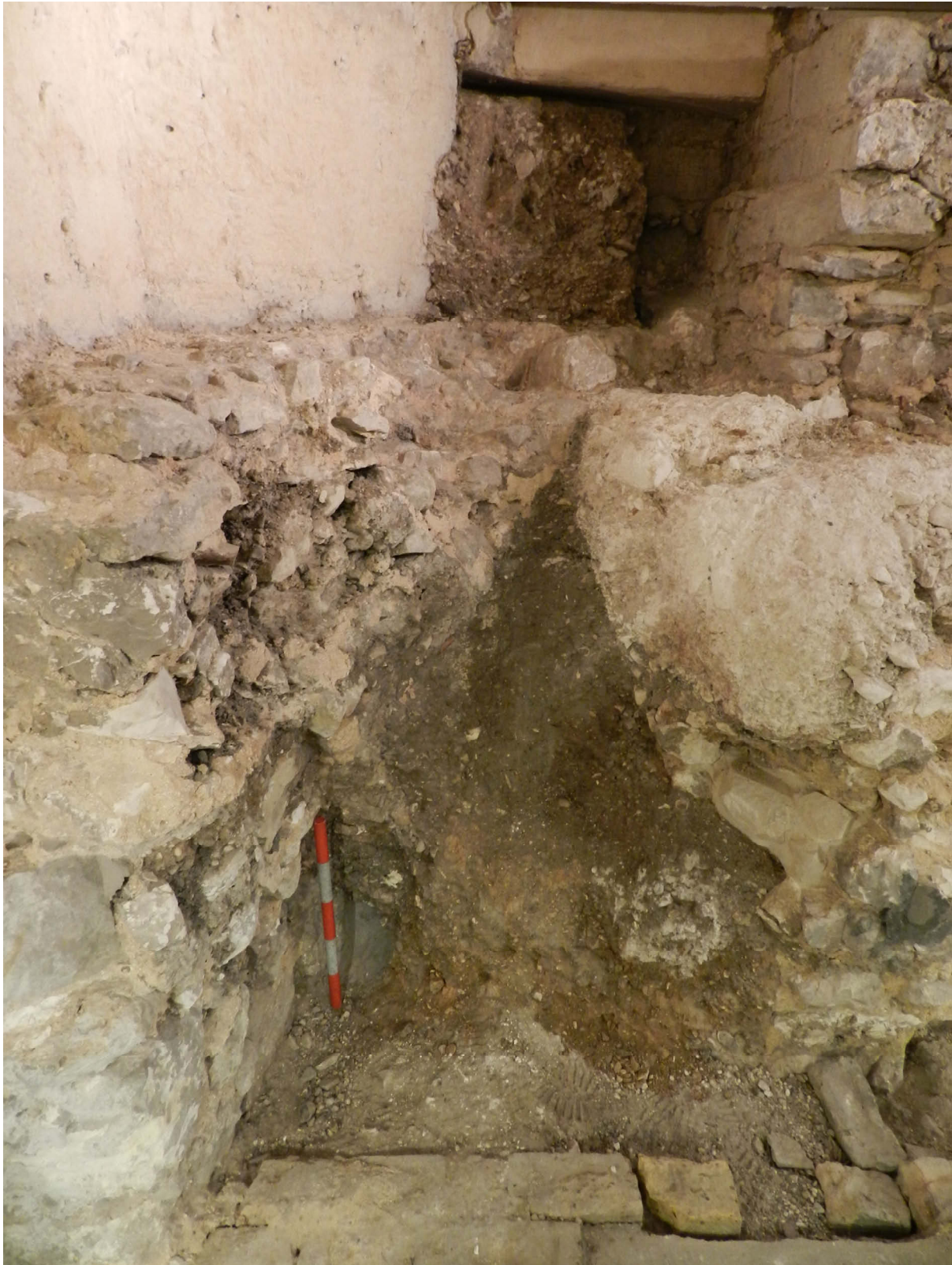
Fig 12 Humic fill overlying rubble core masonry of the garderobe shaft, looking west
