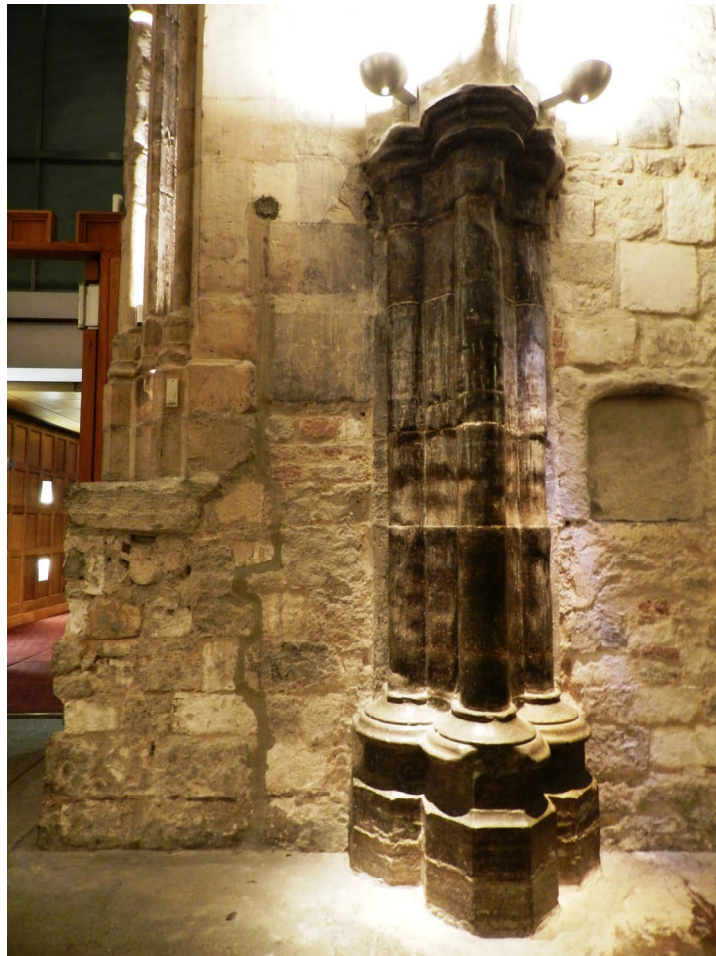
Fig 5 Jamb of east door to the East Crypt, Purbeck clustered shaft and lavabo, looking east
