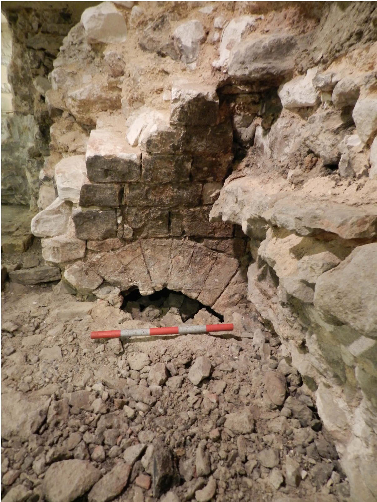
Fig 13 The voussoirs of the garderobe cesspit with the soakaway chamber and vaulting, looking south
