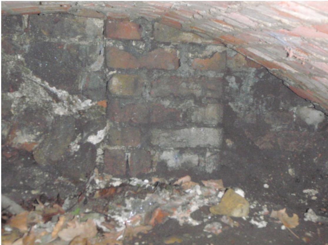
Fig 6 The rear of tomb 119, showing the graveyard wall foundations and the brick column which supports railings, looking east
