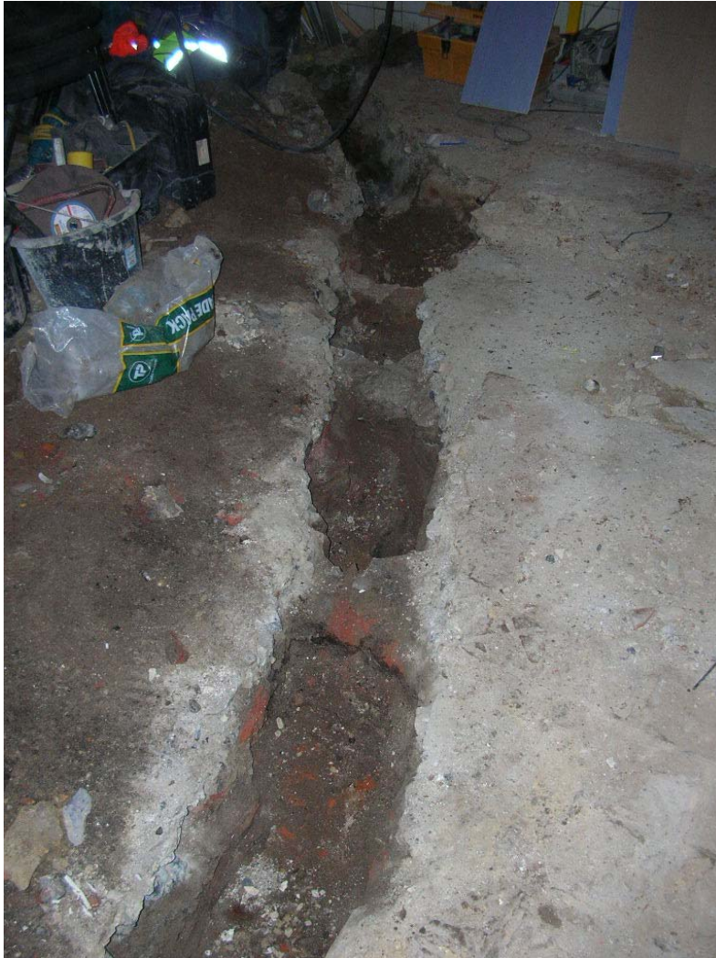
Trench 3 with brick footings looking north
