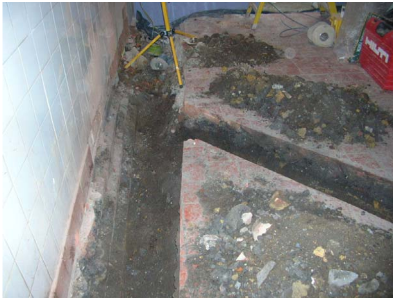
Trench 2 and junction with Trench 1 looking south-east
