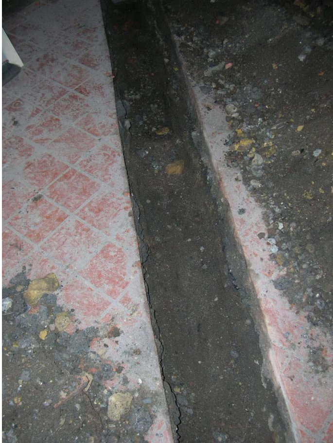
Trench 1 looking south-west
