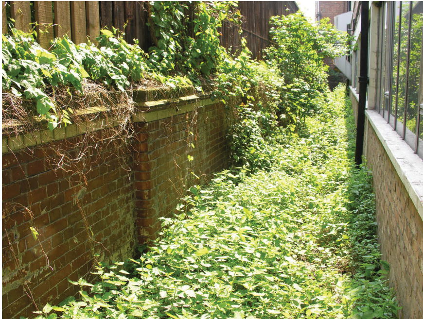
Fig 5 Structure 2 on left and Building 4 on right, view to south
