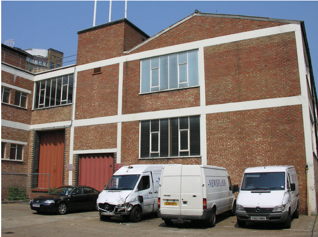
Fig 10 View looking north at the loading bay side of Building 5
