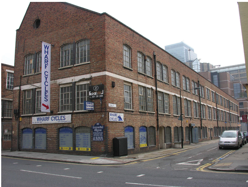
Fig 7 View looking north-east at Building 4, showing the Westferry Road frontage (left) and the Cuba Street frontage (right)
