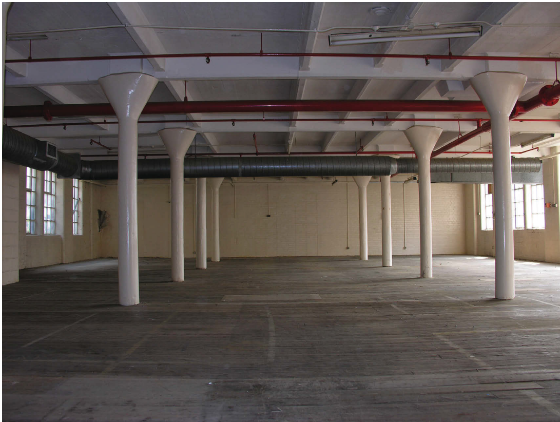
Fig 8 First floor of Building 4 , view to east
