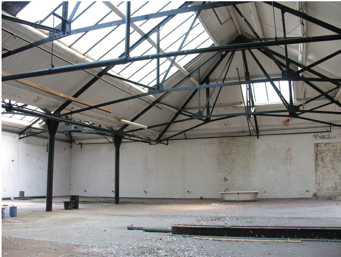
Fig 9 Second floor of Building 3, view to east
