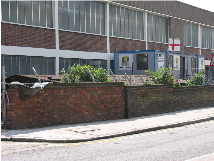
Fig 4 Structure 1 on right hand side, view to southeast
