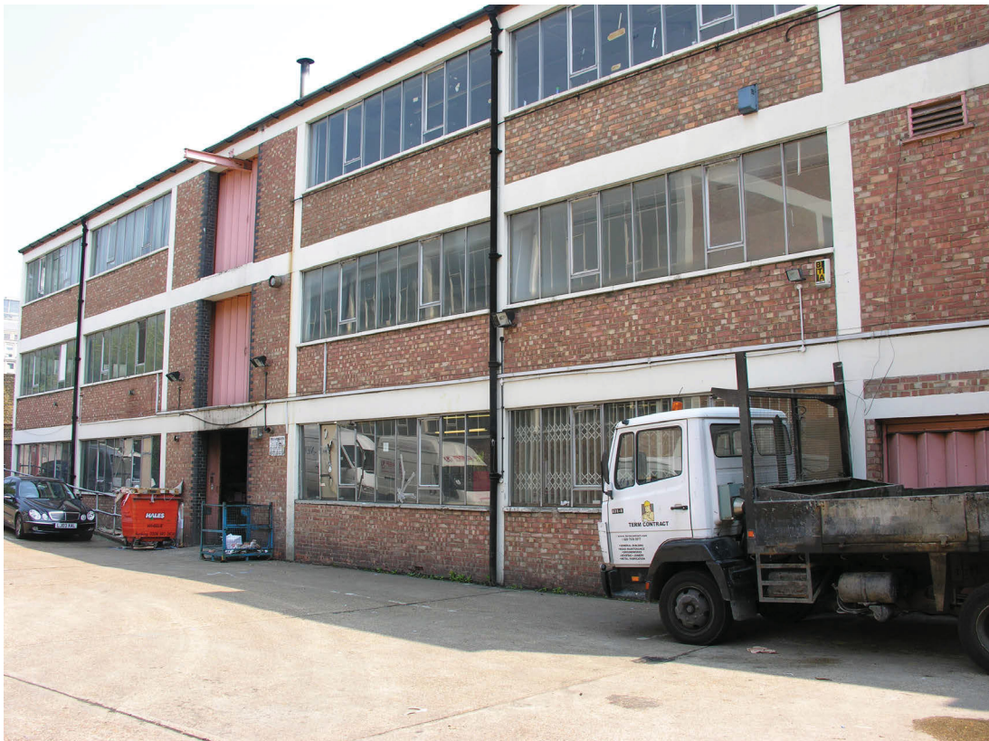
Fig 11 View looking north-east at the main facade of Building 6.
