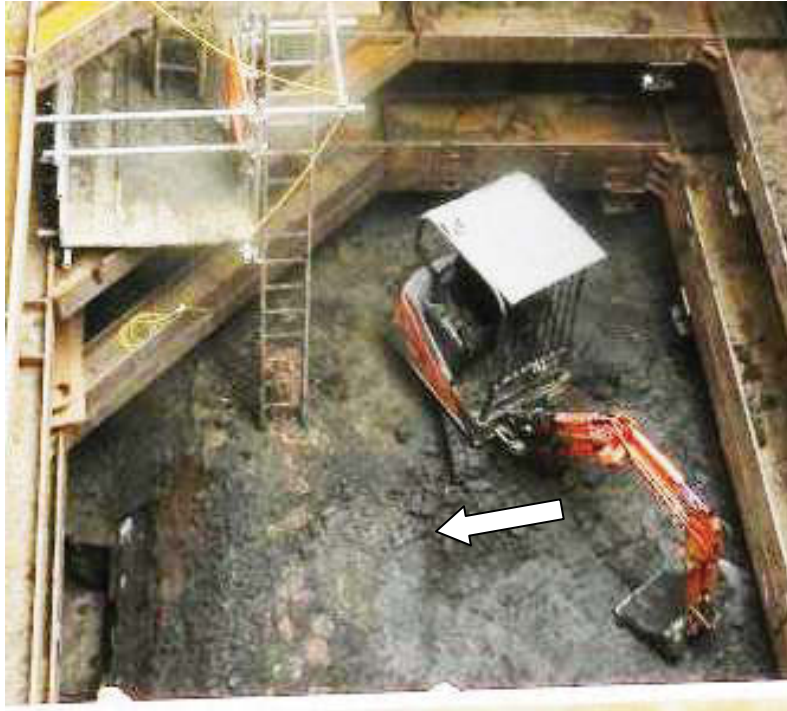
Photo 4 detail of above photograph – Ham Sewer indicated by arrow
