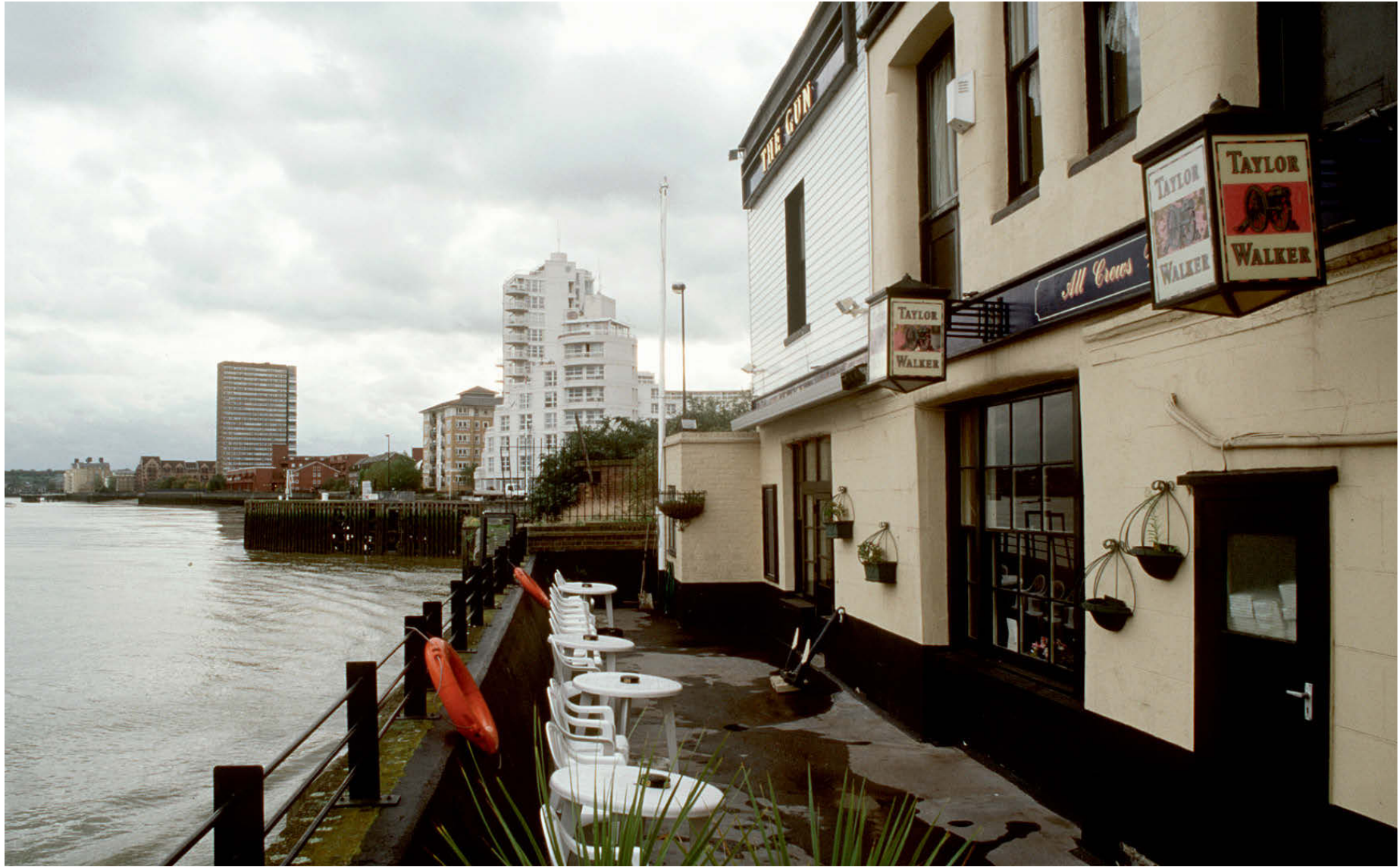
Figure 19. The riverfront of The Gun, looking south-west
