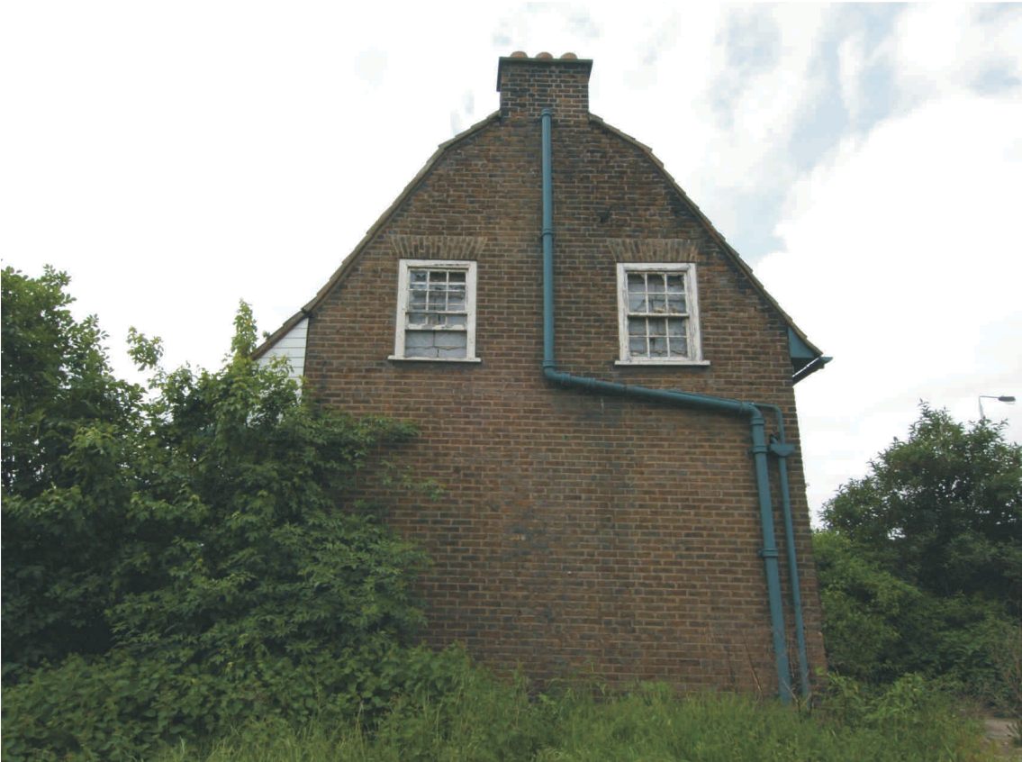
Fig 4 View of north-eastern elevation, Building 1 (Image ref no: 141/06/032)
