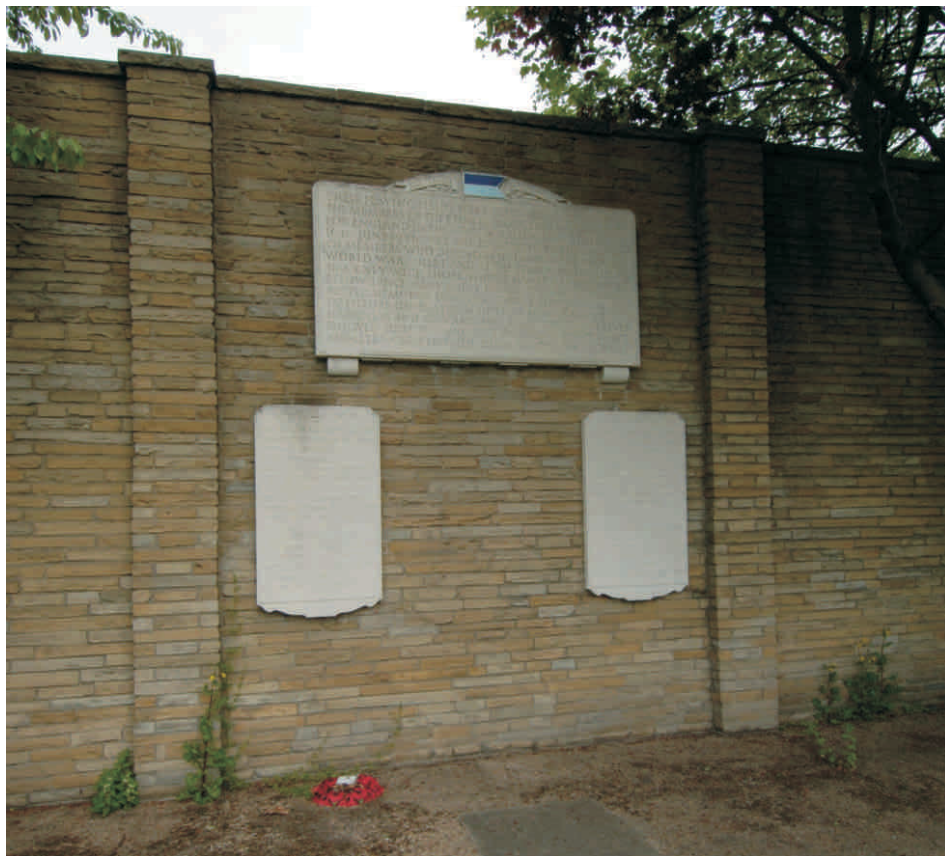
Fig 11 General view of Structure 2 (Image ref no: 141/06/020)
