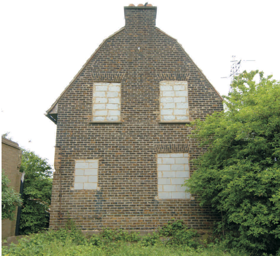
Fig 3 View of south-western elevation, Building 1 (Image ref no: 141/06/036)
