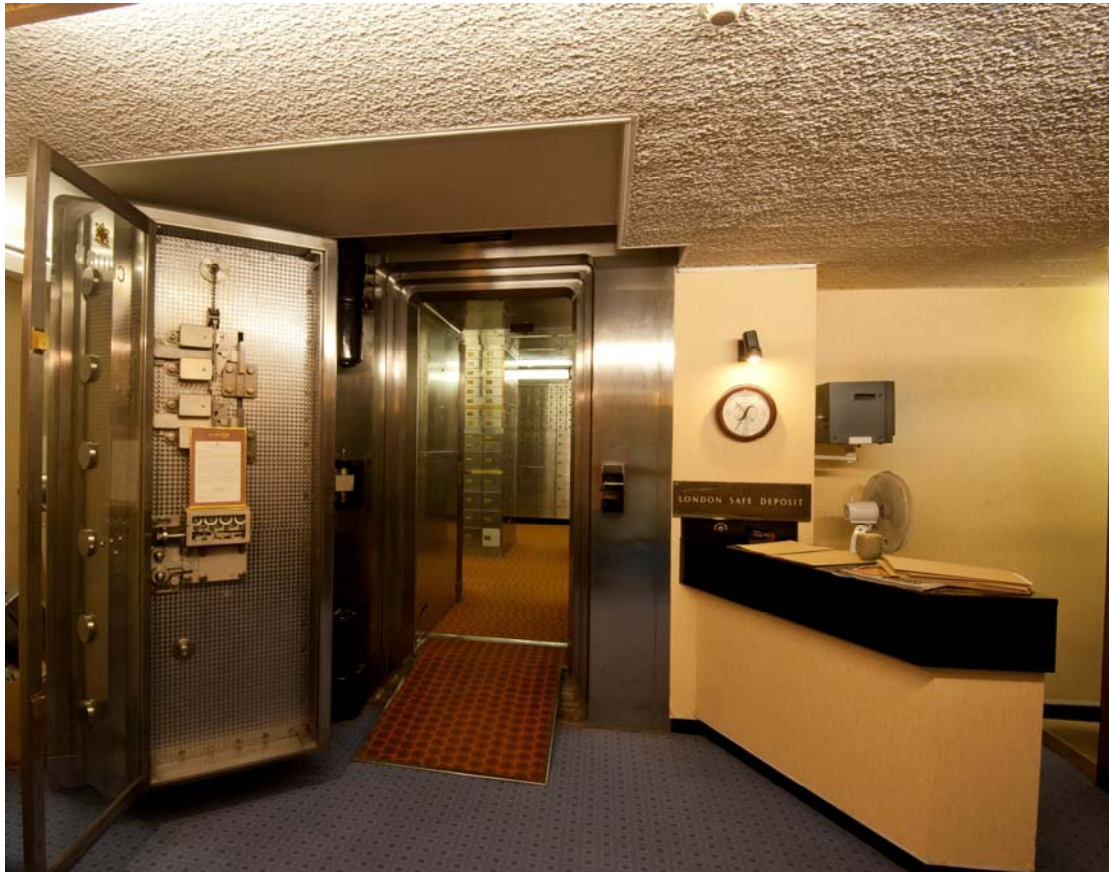
Figure 4. Strong room entrance and 20 ton door, looking south-east.
