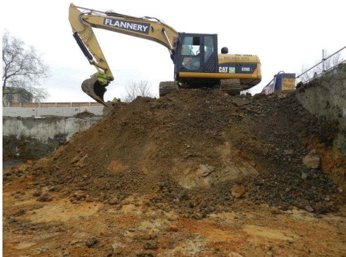
Photo 14 bulk excavation of south area of shaft
