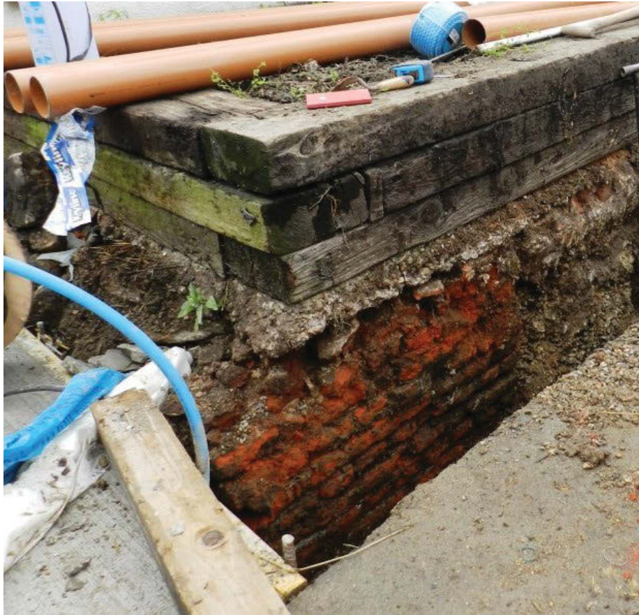
Photo 7 Wall made of Tudor-style bricks [331] beneath the raised bed west of City Farm offices
