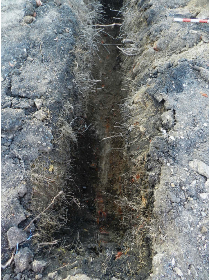
Photo 3 Trial Pit 3 looking south, on the east side of the craft building. A nineteenth-century brick coal cellar dug through landfill deposits of similar age, at 109.1m ATD
