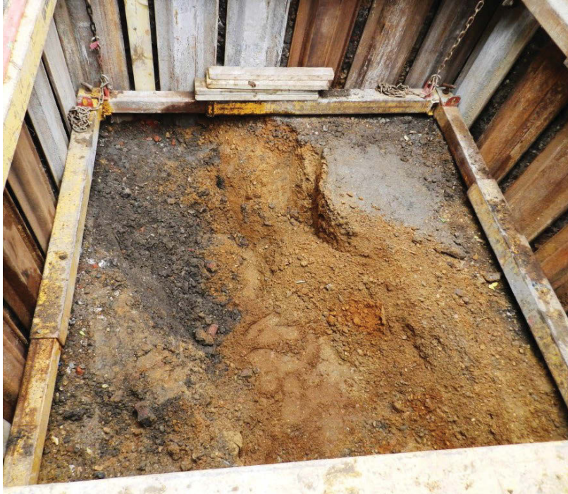
Photo 10 Full depth of temporary drainage manhole. Coal-ashy fills [322] continuing
