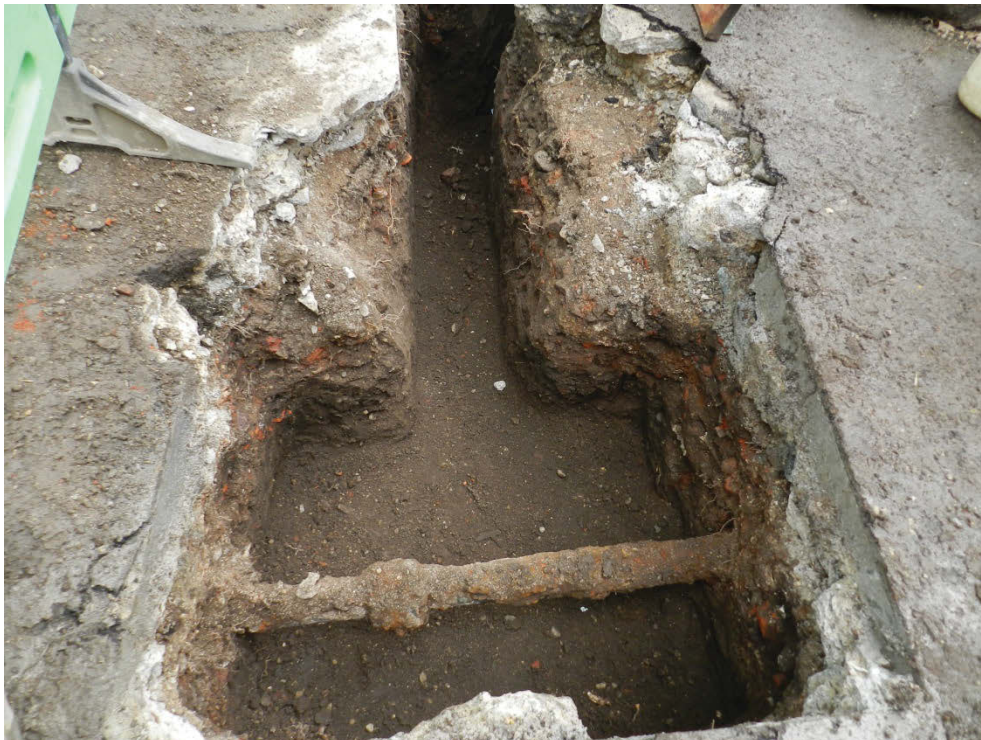
Photo 11 Water main, initial trench to connect to existing pipe, subsequently enlarged
