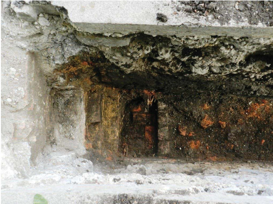
Photo 19 Culvert [336] (north is top) East trench
