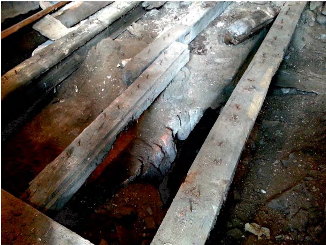
Fig 15 Trench B7, looking north, showing brick vault beneath existing floorboards
