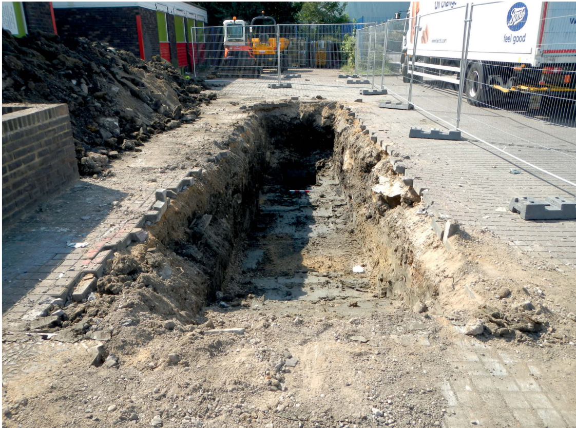
Fig 8 Trench 4; general view; facing W
