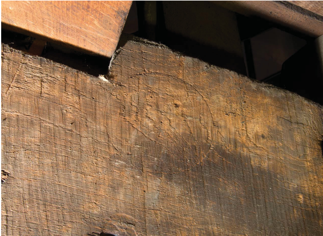
Fig 15 close up of a large historic oak rafter of St Pauls cathedral type reused in recent additional truss 22b over the portico roof. The faint outline of part of a compass drawn daisy wheel, possibly a 'witch mark' is visible cutting through the pit saw marks
