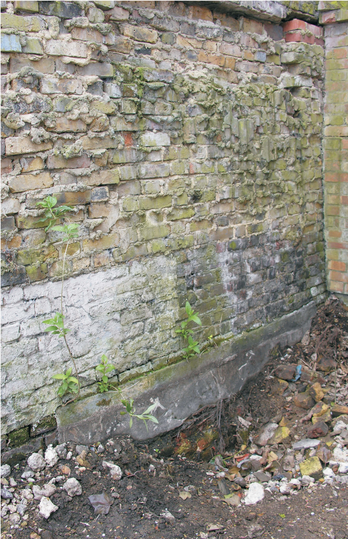
Fig 4 Photograph of 19th century wall
