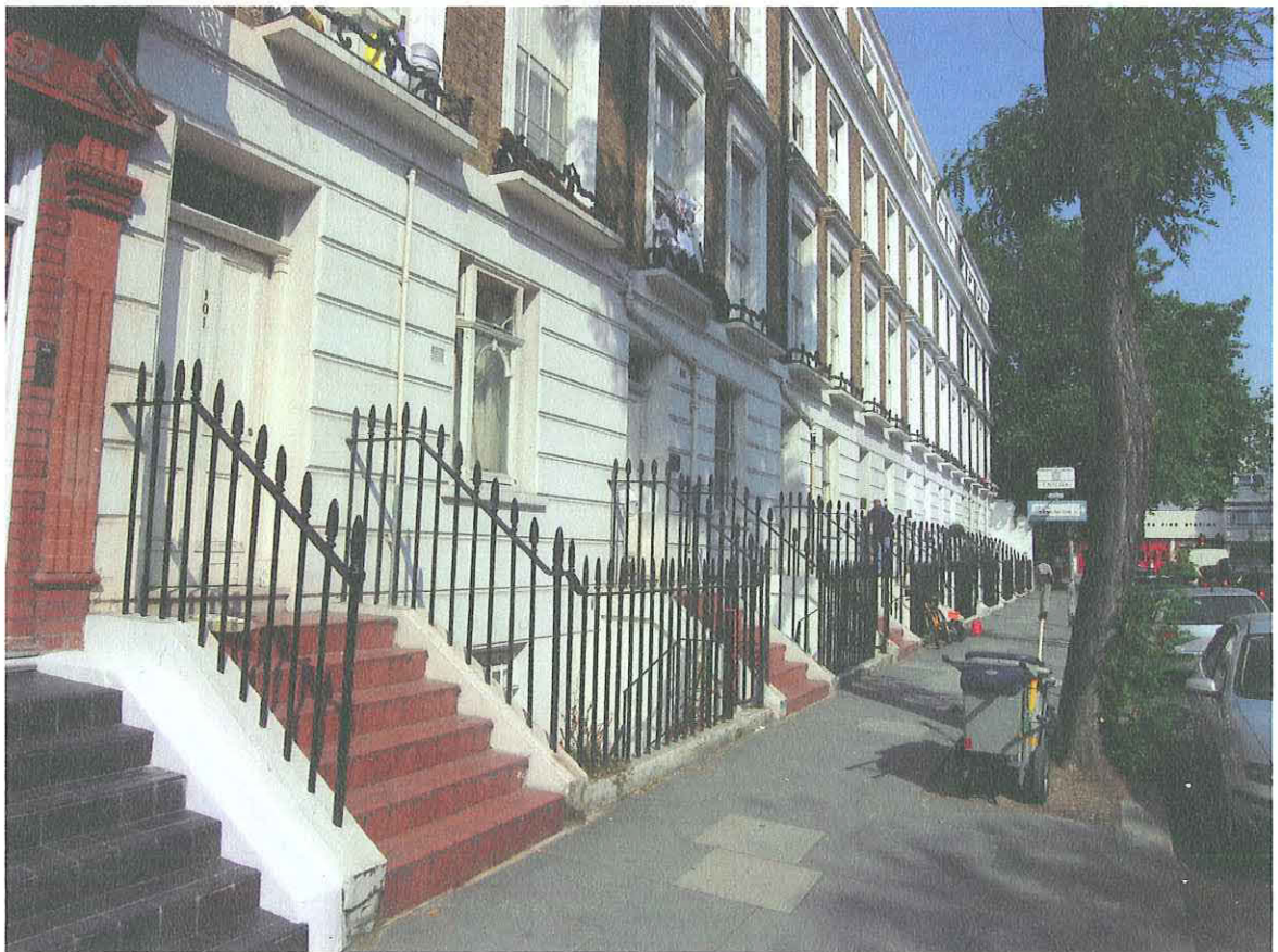
Fig 5 Detail of front steps, basement area and railings, looking north-west (MoLAS)
