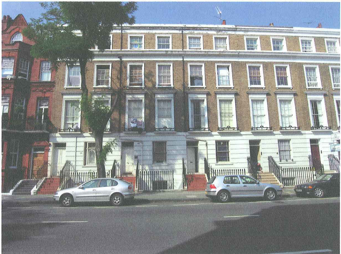
Fig 4 The street front of 101–103 Oakley Street, looking west (MoLAS)
