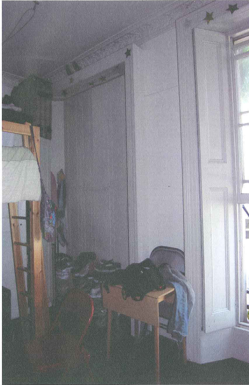
Fig 7 Interior on 1st floor, showing front window shutters closed and open, looking northeast (MoLAS)
