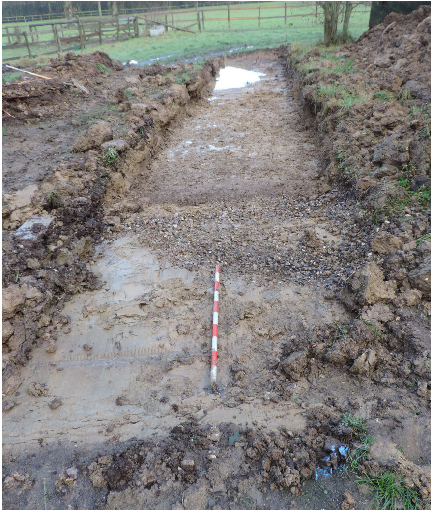
Fig 4: Trench 2, facing north
