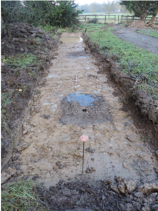
Fig 5: Trench 3, facing west
