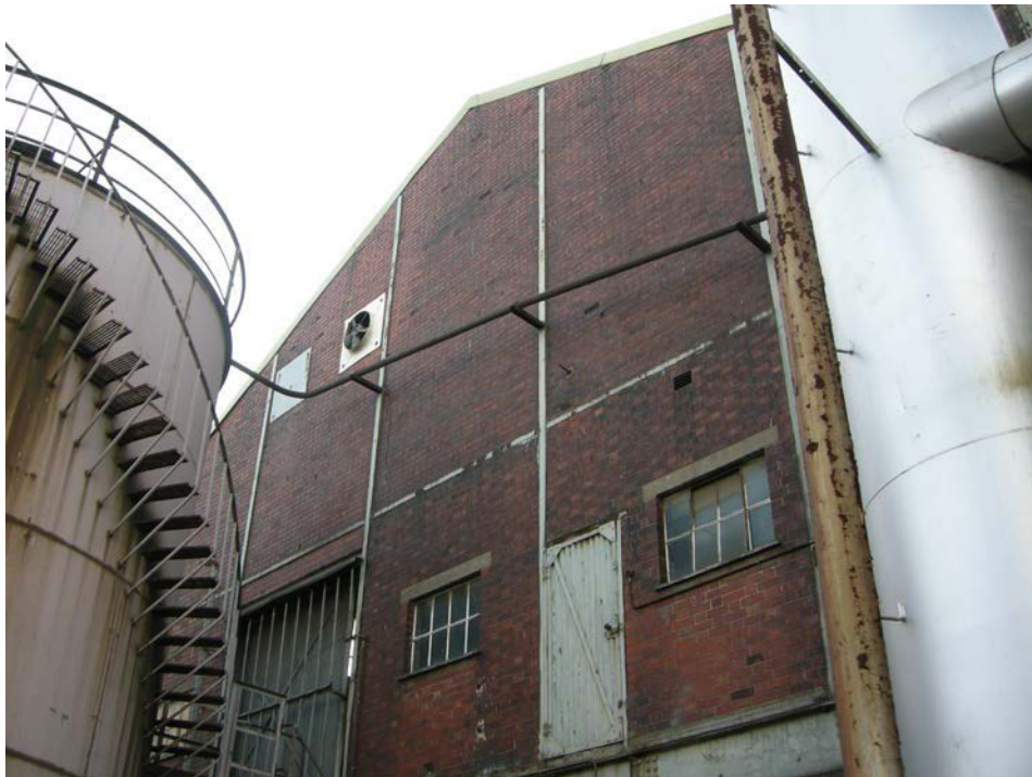
Fig 7 North elevation of the main warehouse (MOLA 2013)
