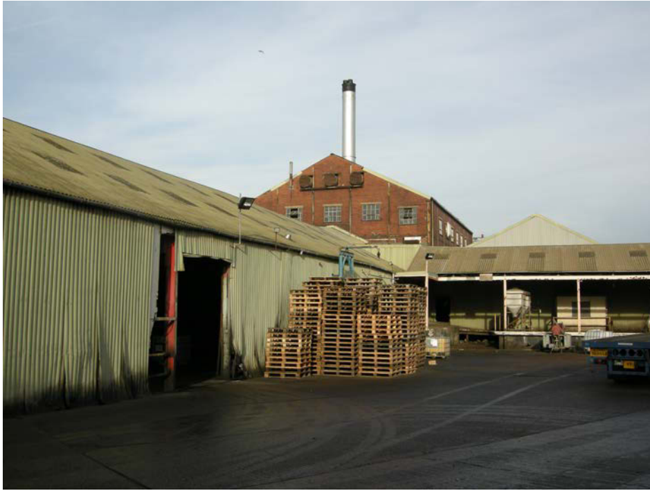
Fig 6 South elevation of the main warehouse (MOLA 2013)
