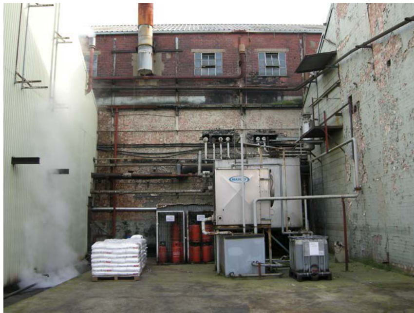
Fig 5 West elevation of the main warehouse (MOLA 2013)
