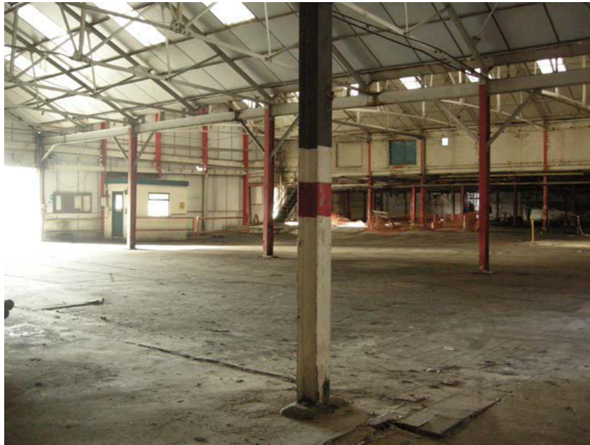
Fig 8 Ground floor looking towards main warehouse (MOLA 2013)
