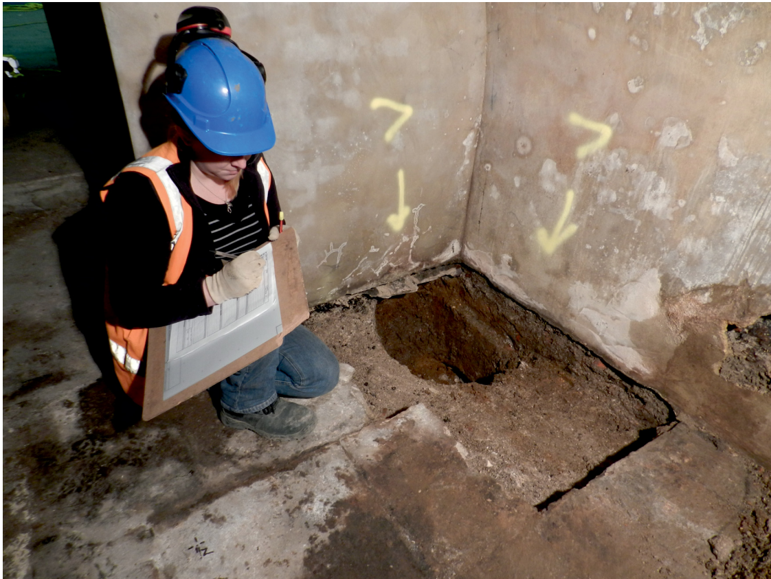
Fig 13 Photograph of test pit 7 (looking south east)
