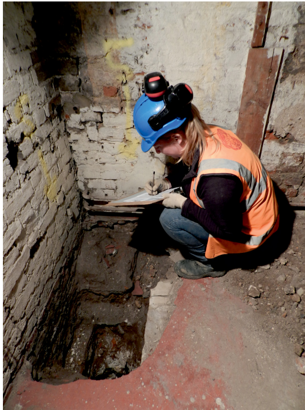
Fig 11 Photograph of test pit 5 (looking west) showing possible remains of chalk wall showing under the foundations of the current building
