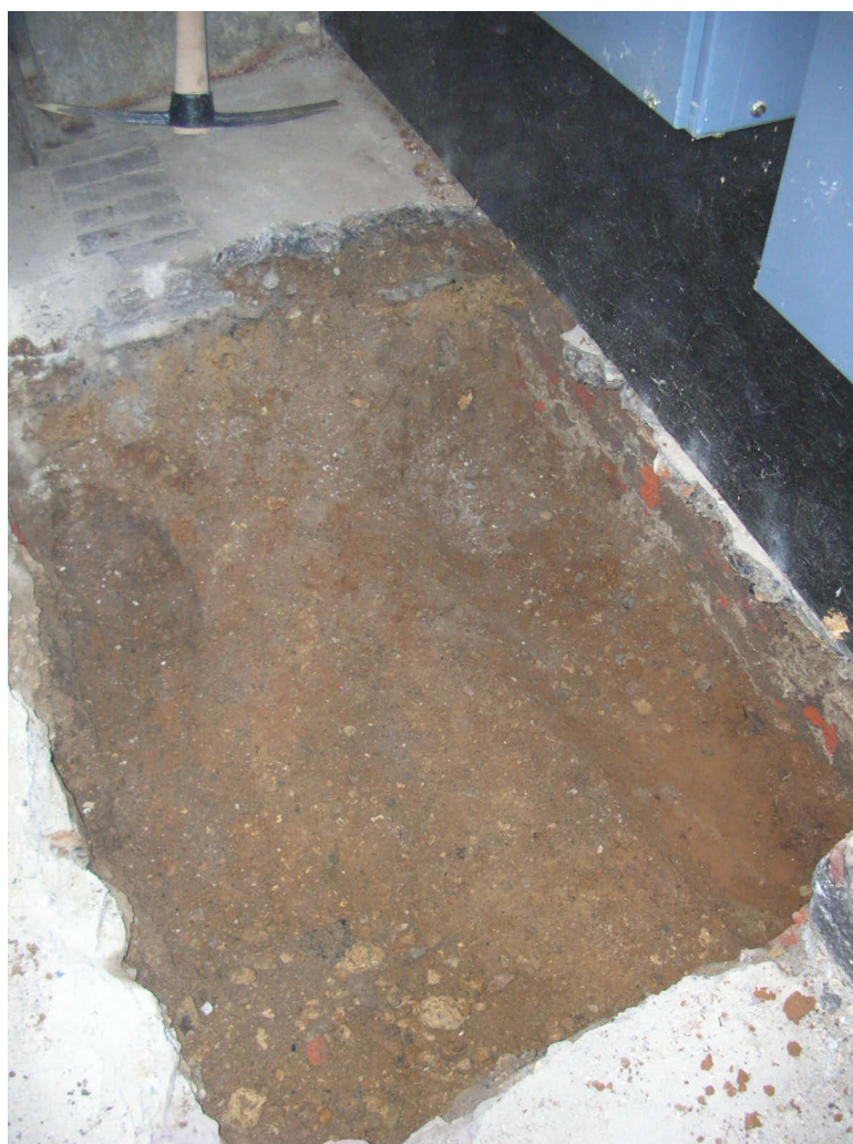
Trial pit B looking east
