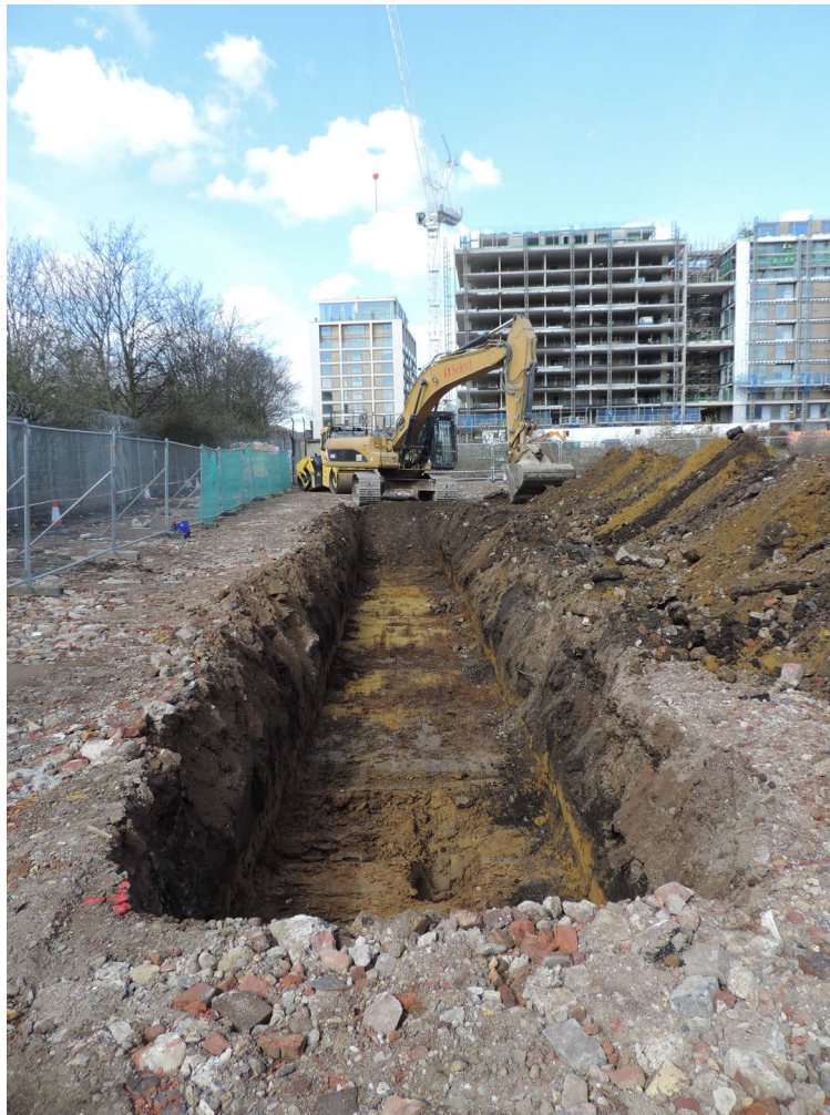
Photo 1 Trench 1 looking NW
