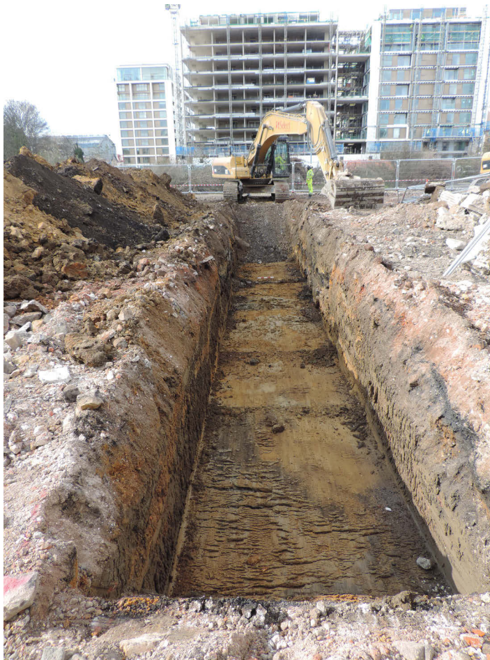
Photo 3 Trench 3 looking NW
