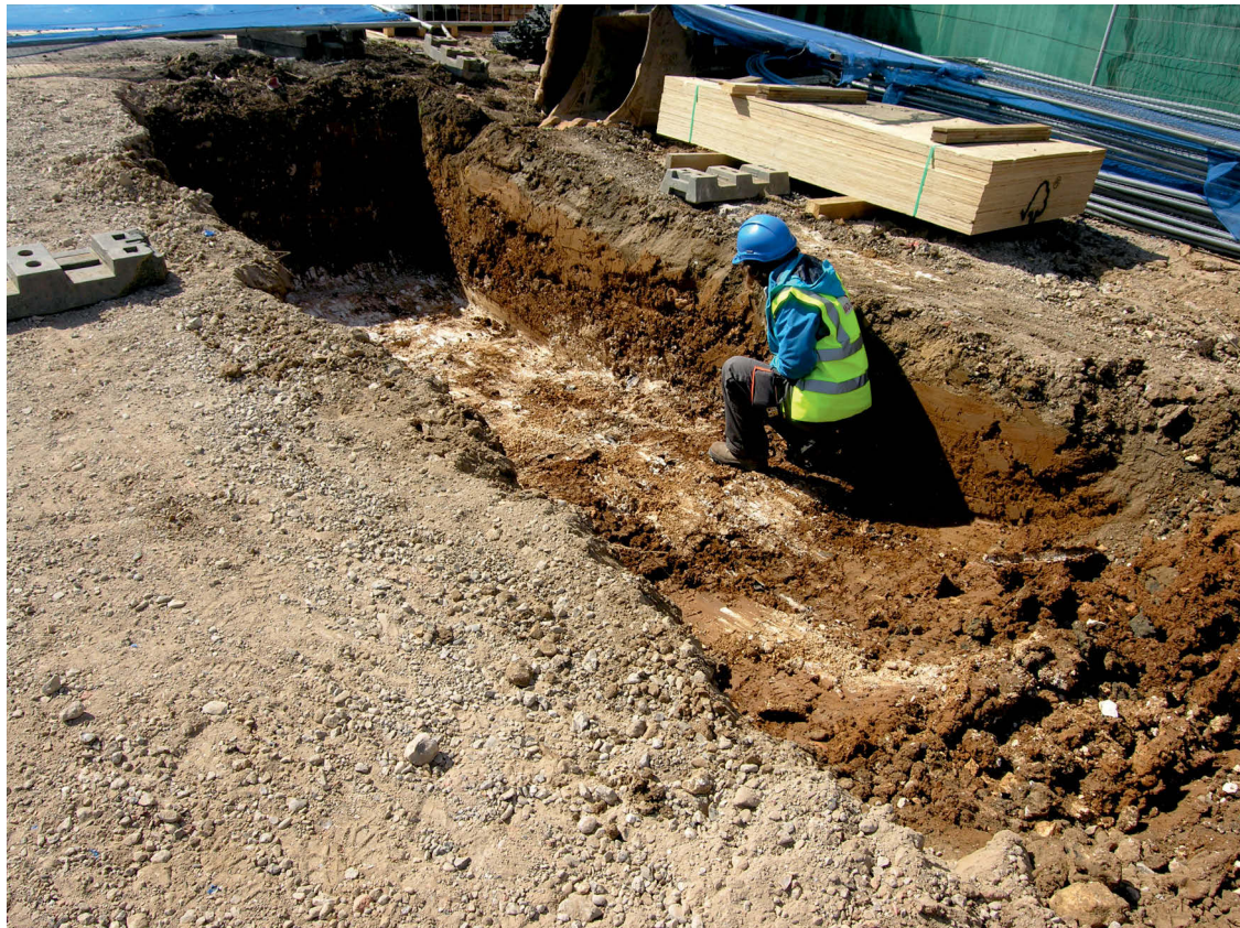
Fig 8 Photo of trench 6
