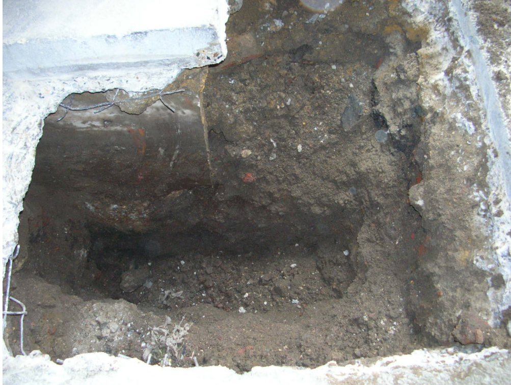
TP17 looking south
