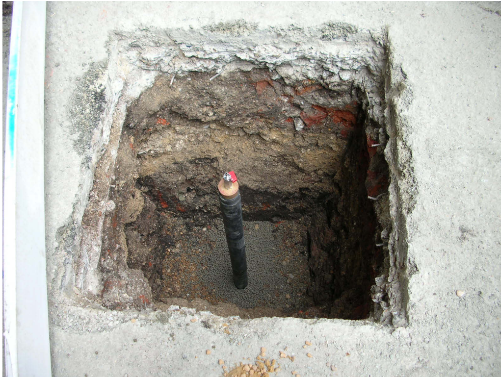
WS pit 6 looking west
