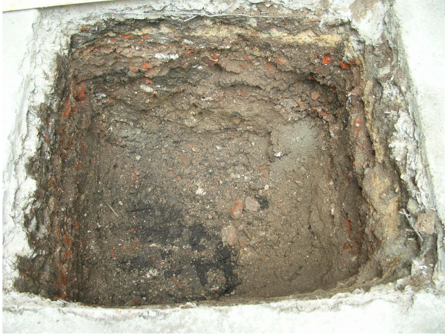
Soakaway pit looking west
