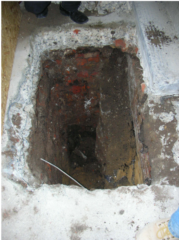
TP15 looking east
