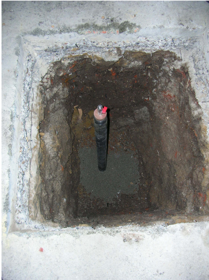
WS pit 5 looking west
