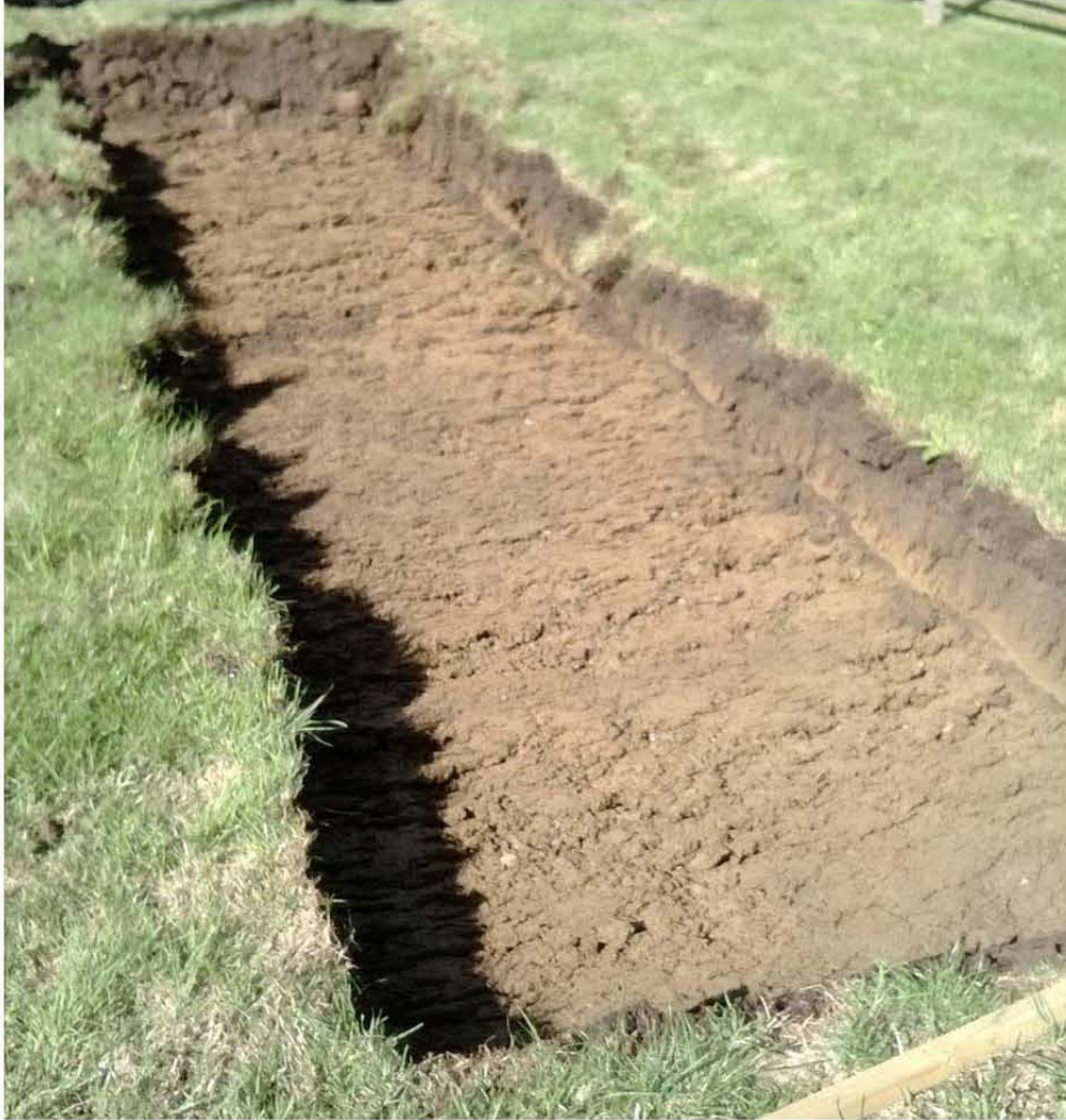
Fig 5 Trench 3 Facing south-west
