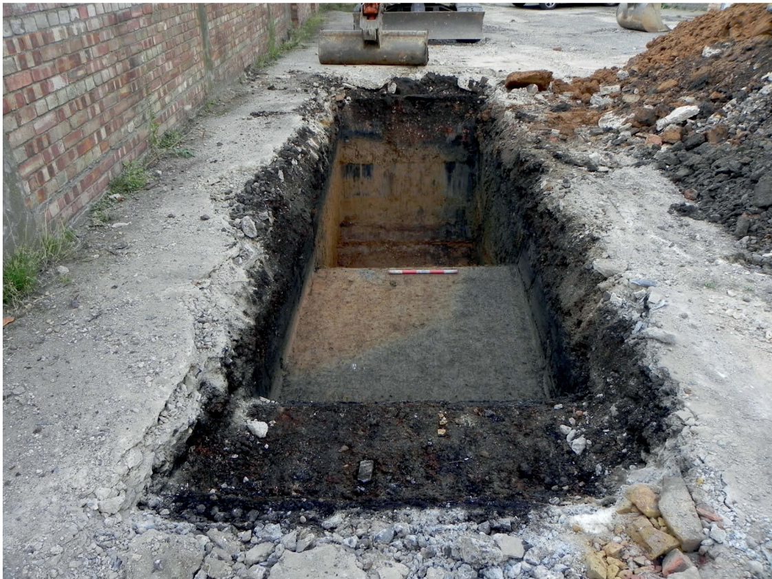
Fig 9 Trench 11 facing west
