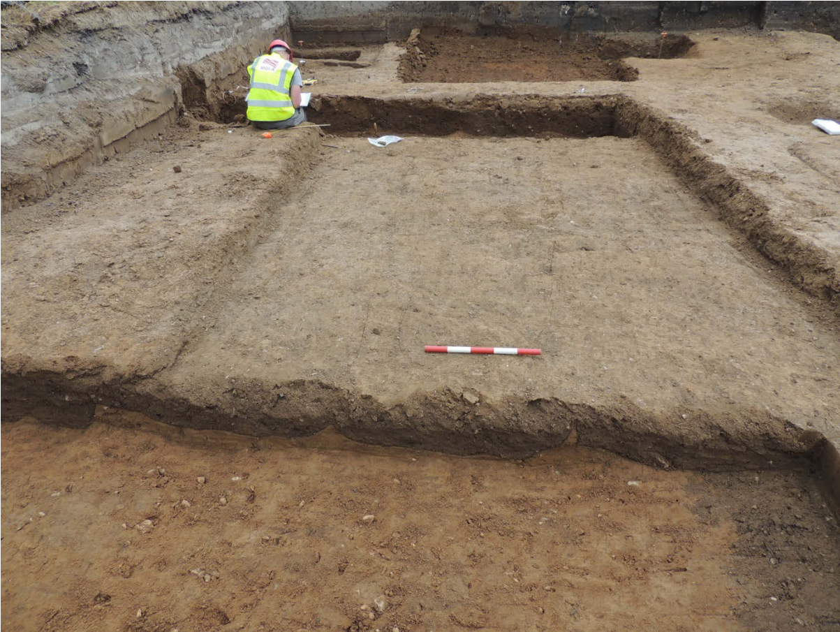
Fig 22 Trench 22 looking south, bedding trenches [3375], [3378], [3380] and [3382]
