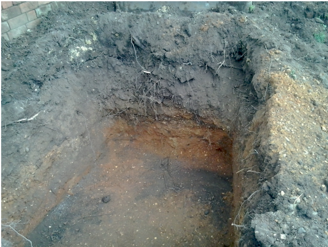
Fig 4 Excavation for the Sewage Pump facing east
