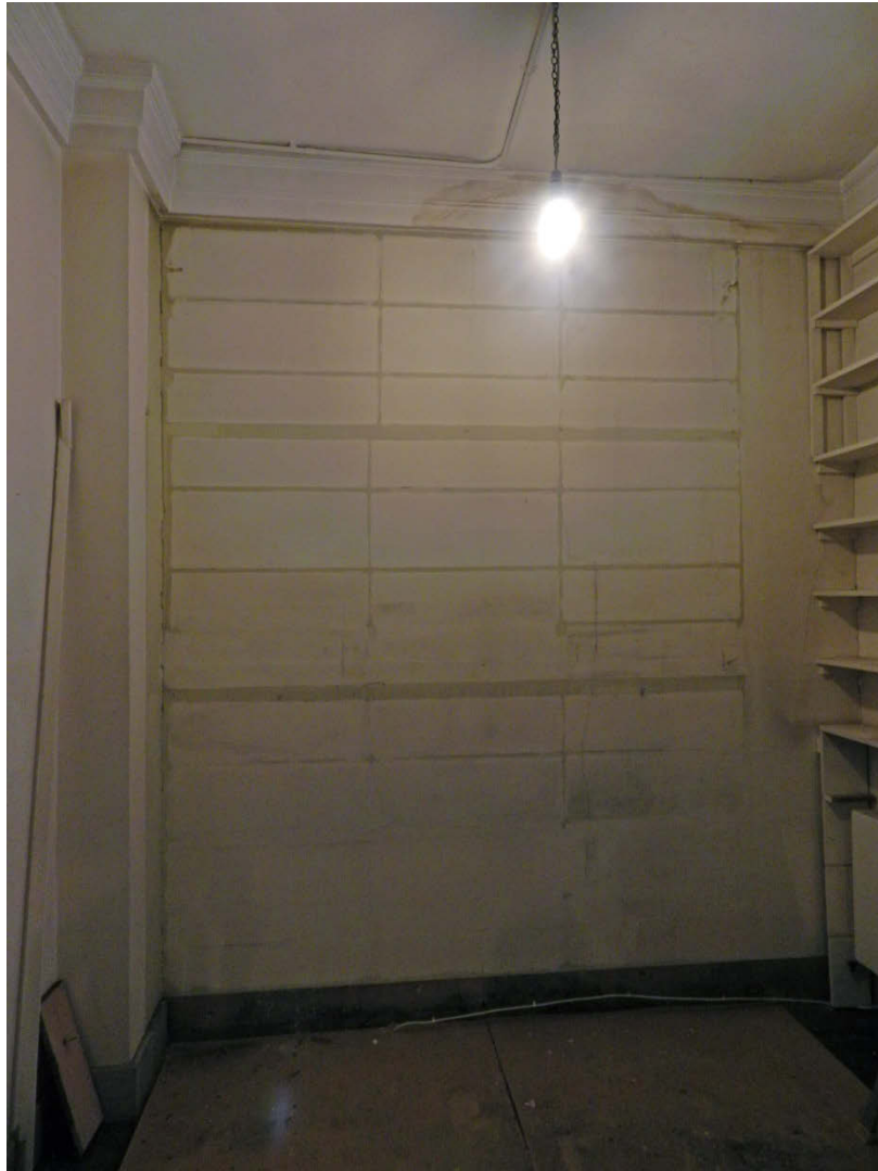
Fig 11 East facing elevation of the tower at first floor level, looking west
