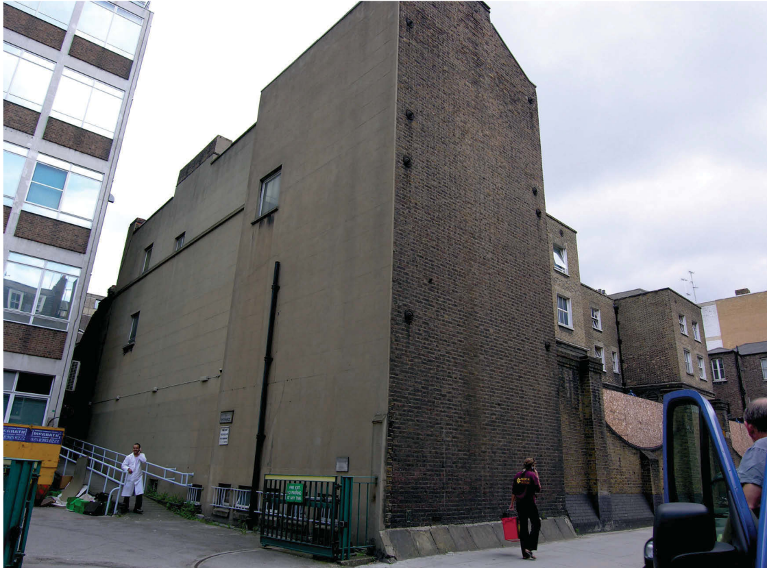
Fig 18 Late 19th-century north range: north elevation and windowless gable end on Cleveland Street
