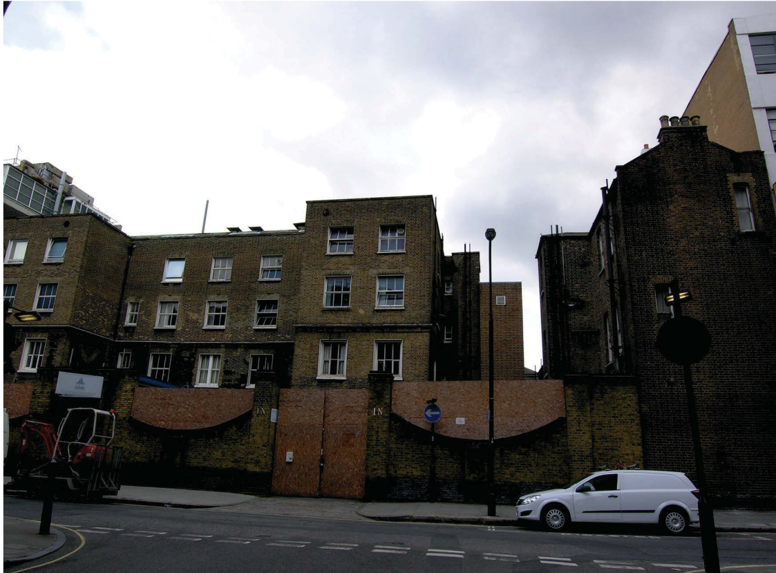
Fig 10 Main front of the 18th-century building (left) and the gable end of the late 19th-century south range (right), on Cleveland Street
