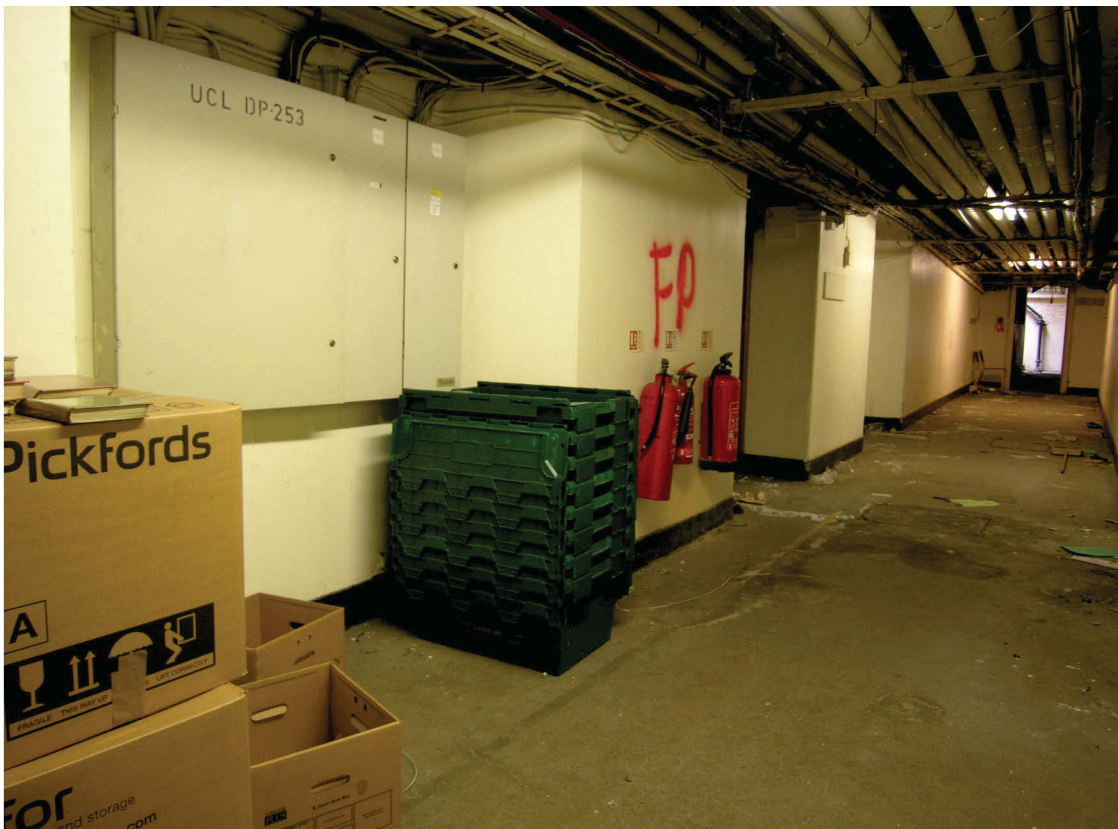
Fig 15 Basement corridor with splayed openings, probably in rear wall of 18th-century building, originally external
