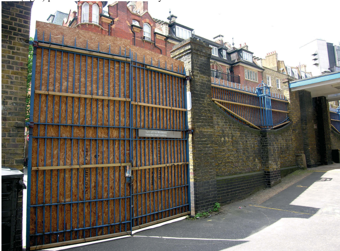
Fig 23 20th-century wall and railings on Cleveland Street frontage and vehicle canopy over main entrance (extreme right)
