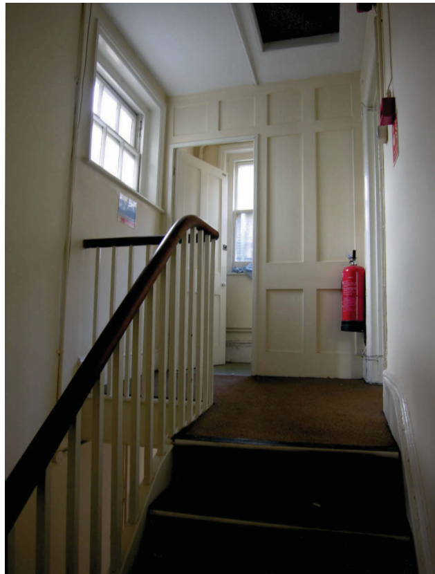
Fig 21 Late 19th-century north range: WC fitted on stair landing at top of east staircase, behind timber panelled partition wall
