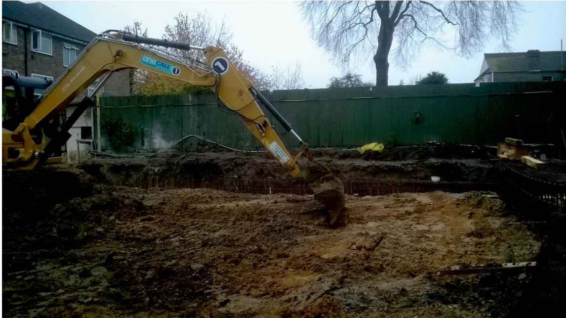
Fig 5 Excavation of central are of site (looking northwest)
