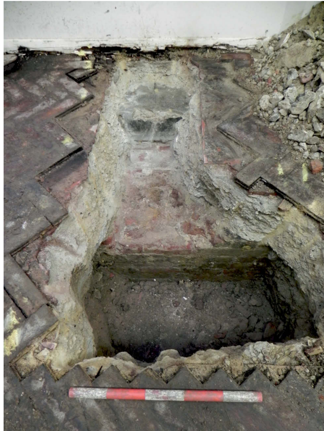
Fig 9 Photograph of evaluation trench 9 showing part of a brick wall foundation of the previous building
