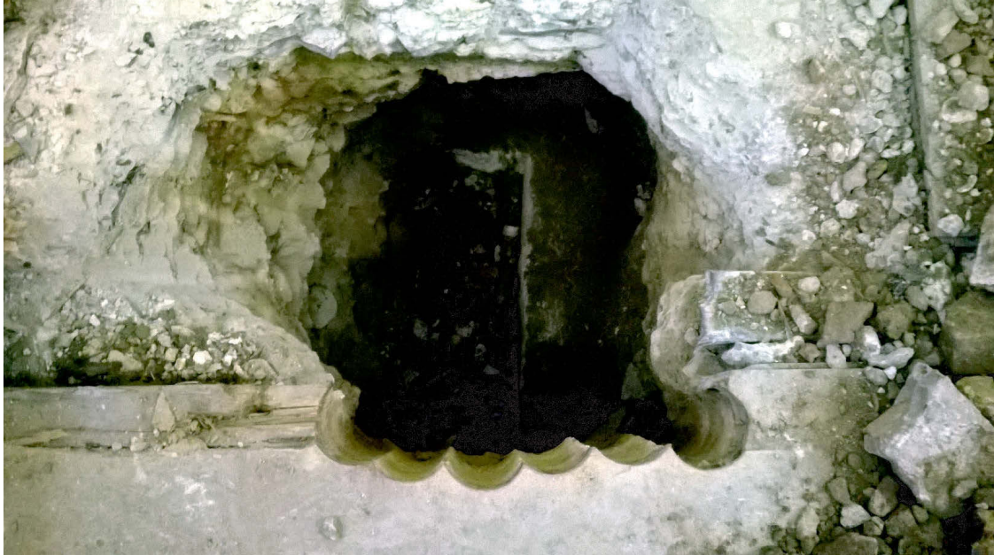
Fig 7 Photograph of evaluation trench 5 showing 20th-century ground beam at the base of the trench (looking north)
