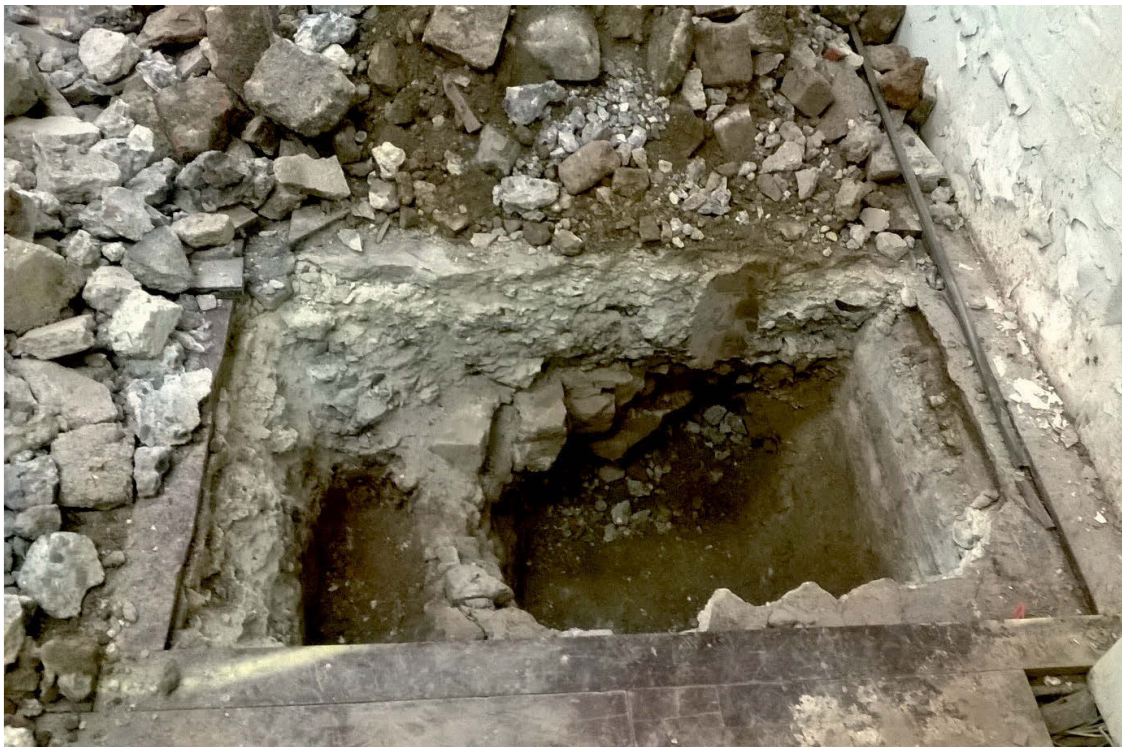
Fig 5 Photograph of evaluation trench 4 showing demolition rubble relating to the building that preceded the present one (looking north)
