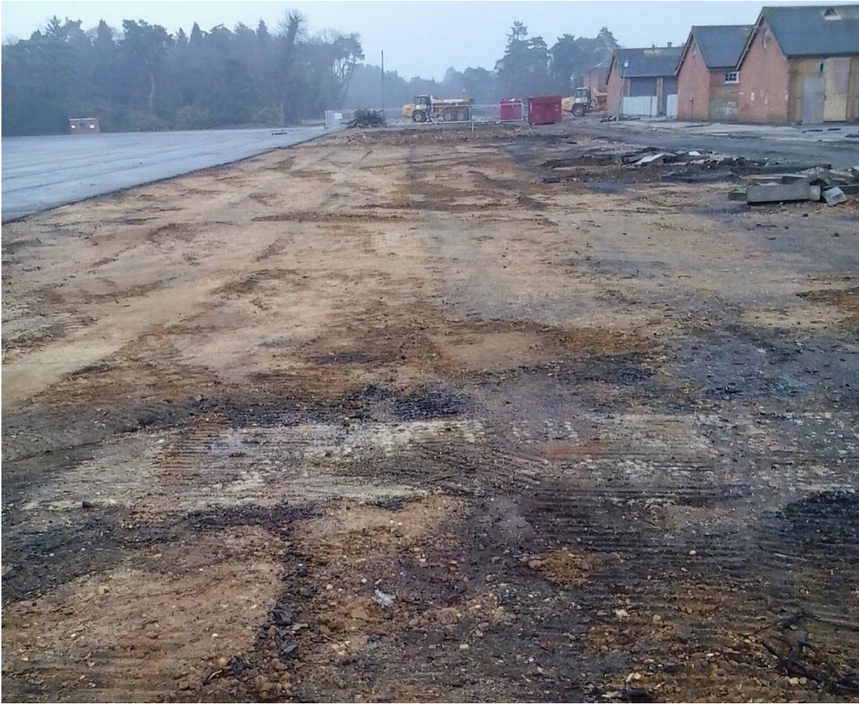
Fig 5 Photograph of Area 3; Facing east
