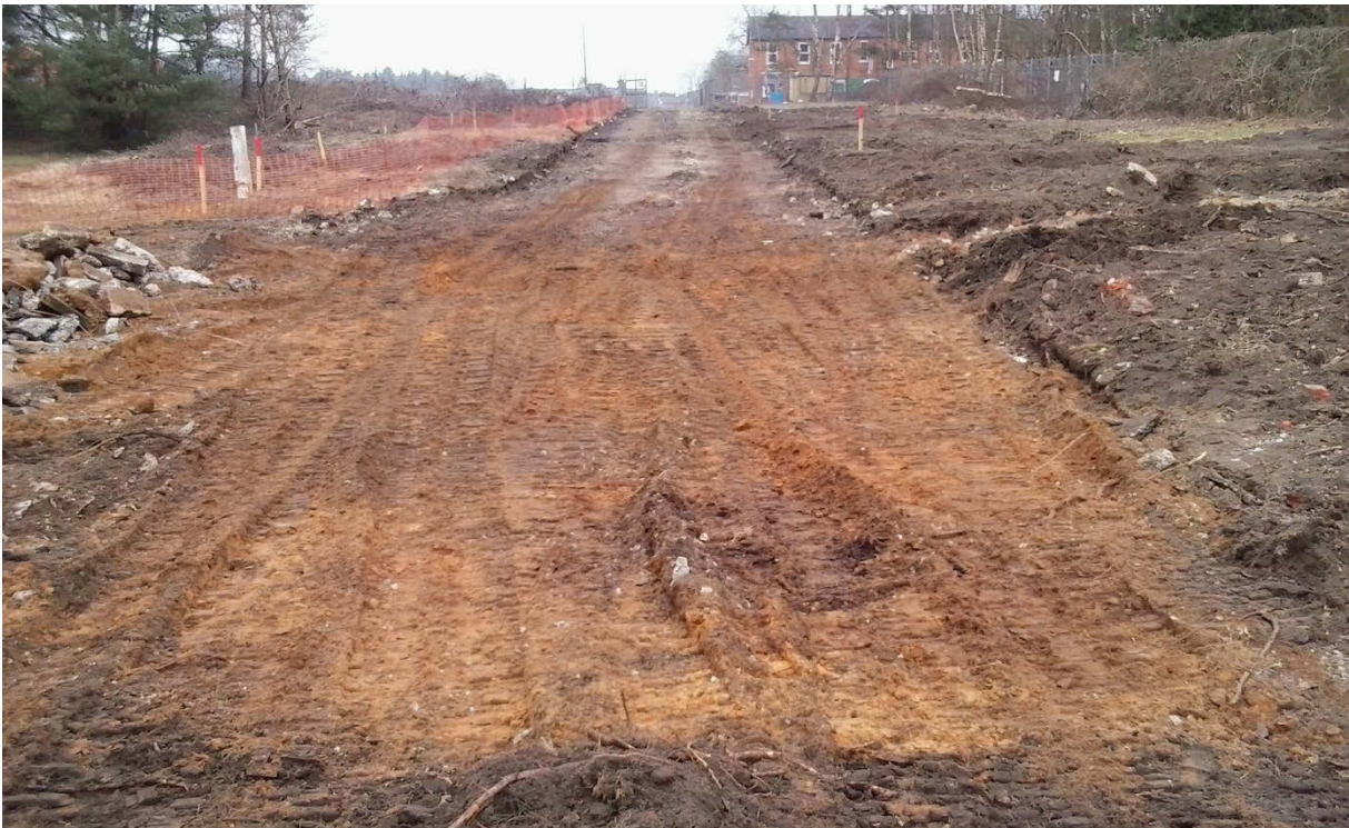
Fig 6 Photograph of Area 4; Facing east
