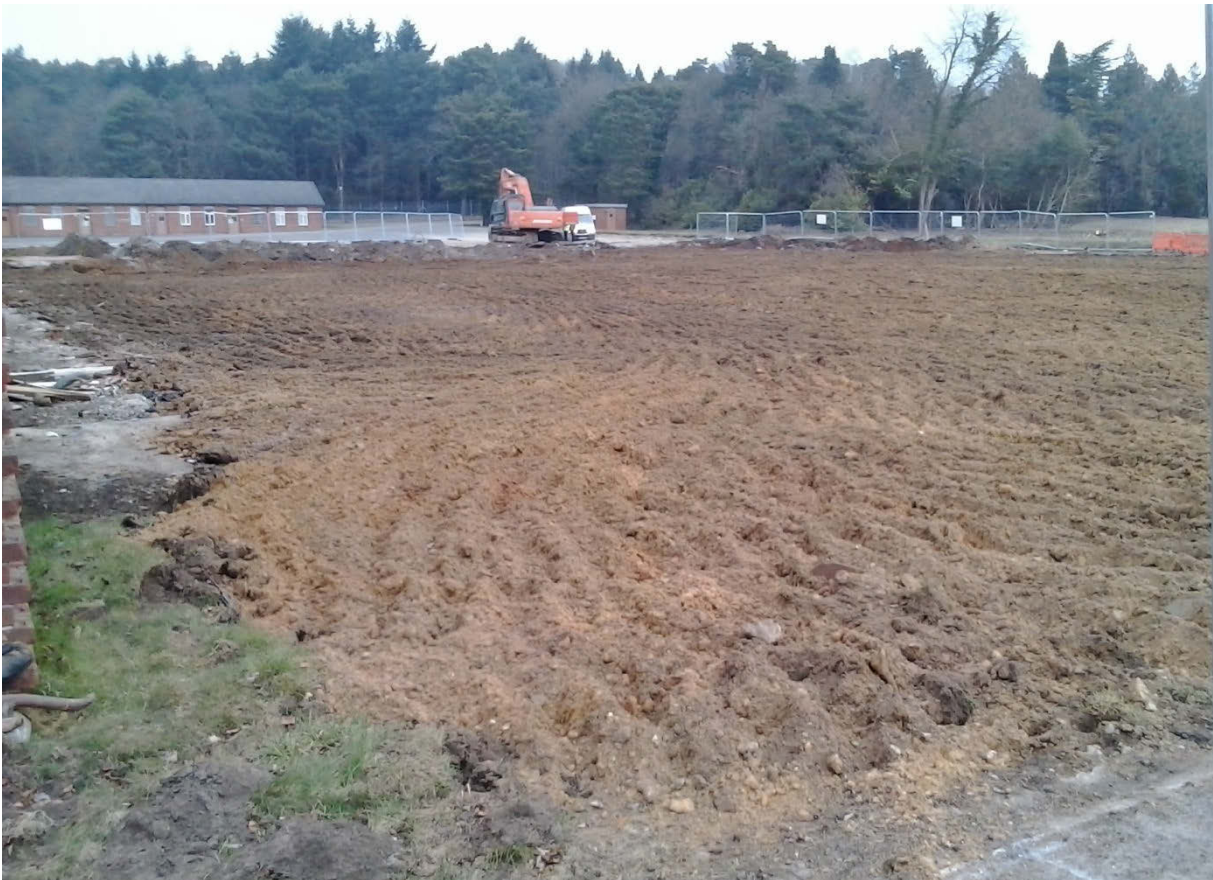
Fig 4 Photograph of Area 2 complete; Facing north-east
