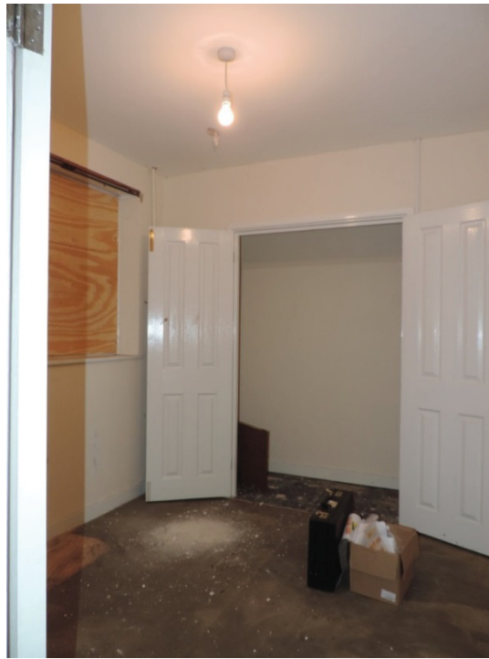
Fig 28 The third bedroom, facing south towards the inserted wardrobe
