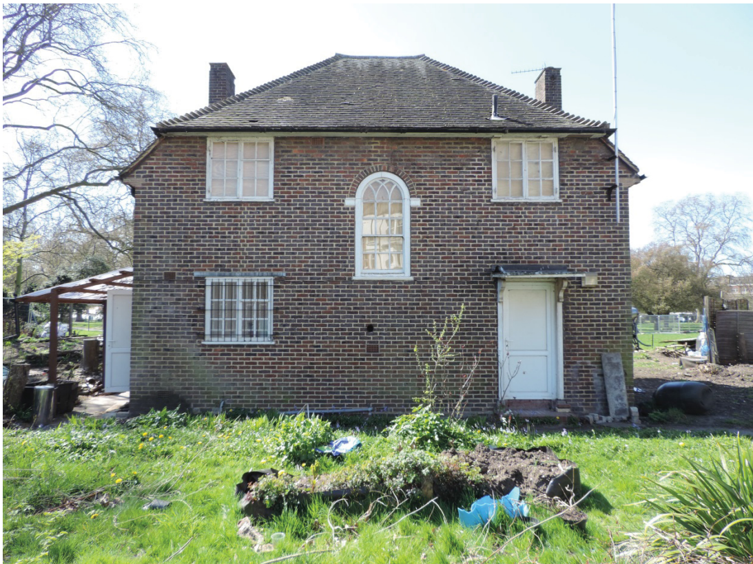
Fig 6 The east elevation of Kennington Park Lodge
