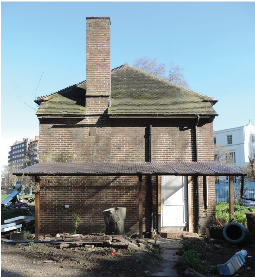
Fig 9 The south elevation of Kennington Park Lodge
