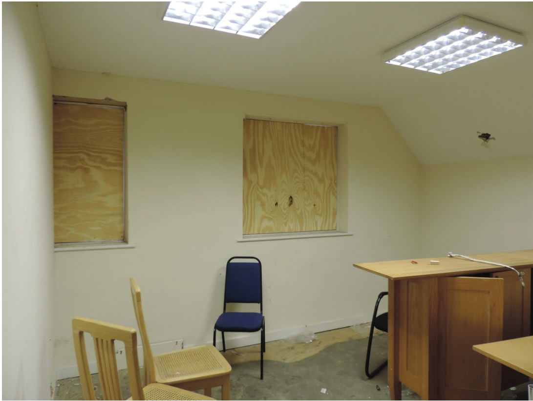
Fig 27 The second bedroom, facing the windows on the west elevation
