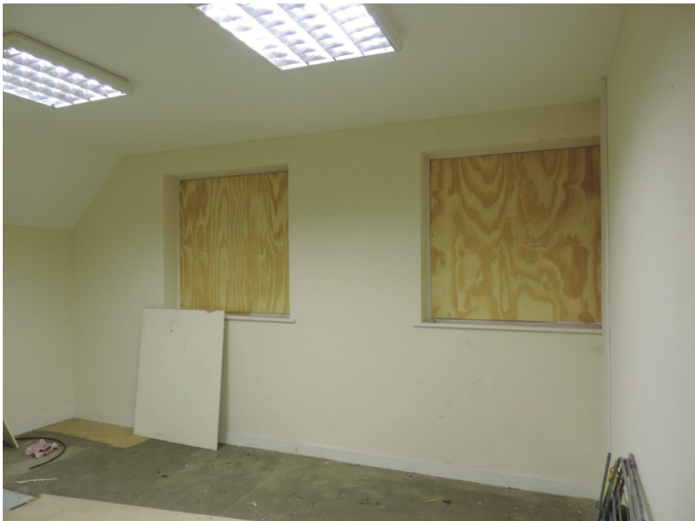
Fig 26 The first bedroom, facing the windows on the west elevation
