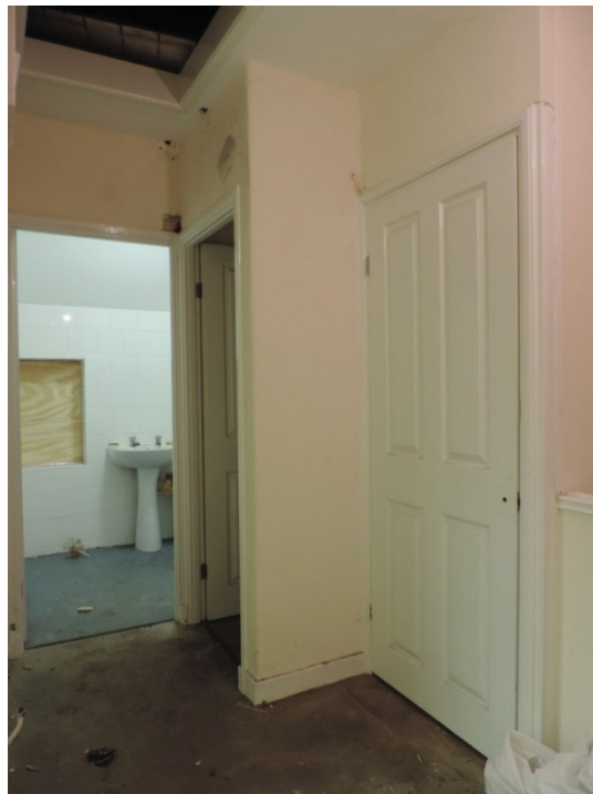
Fig 29 The hall, facing north towards the first-floor bathroom and separate W.C.
