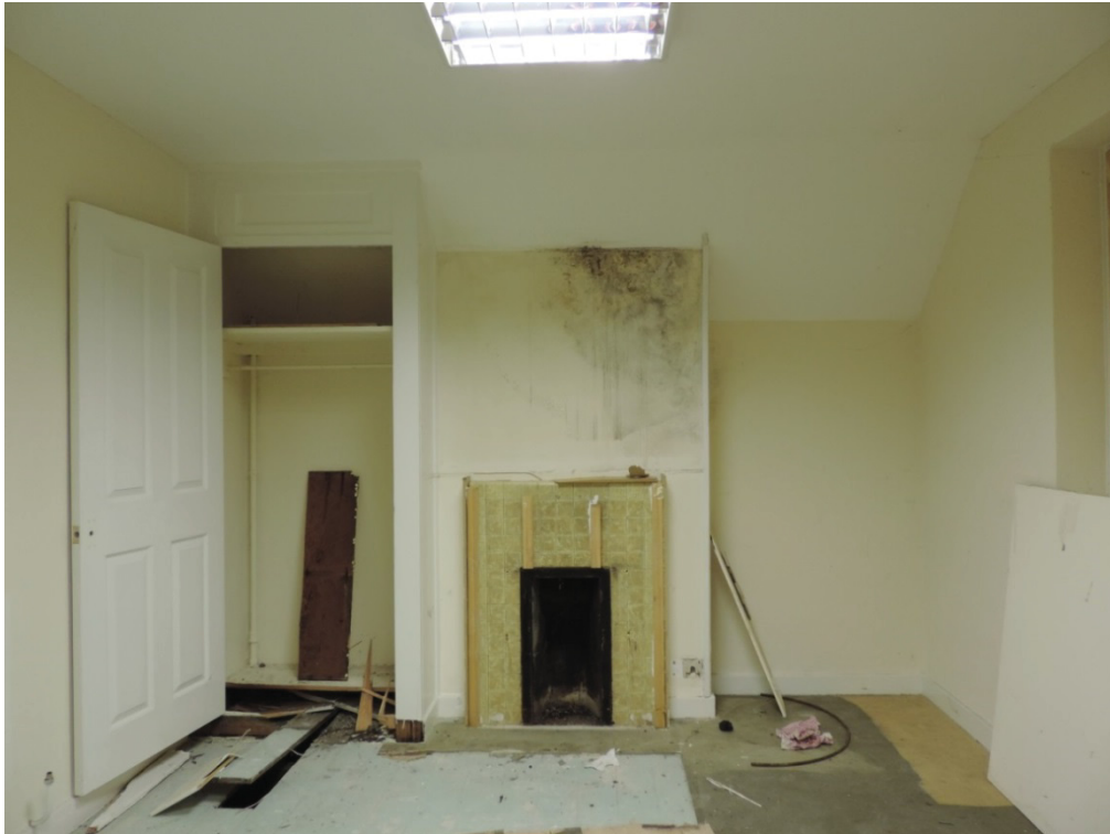
Fig 25 The first bedroom, facing south towards the fireplace and cupboard
