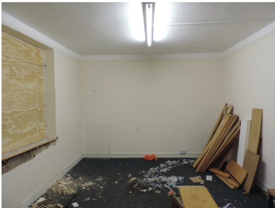
Fig 19 The former parlour, facing north towards the blocked fireplace
