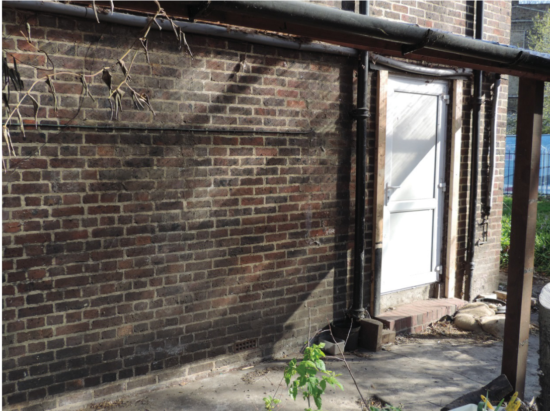
Fig 10 The door opening and contrasting brickwork on the south elevation
