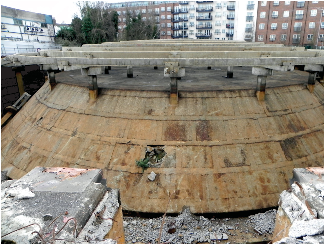
Fig 16 Gas holder 1 (see fig 1) substructure, looking west
