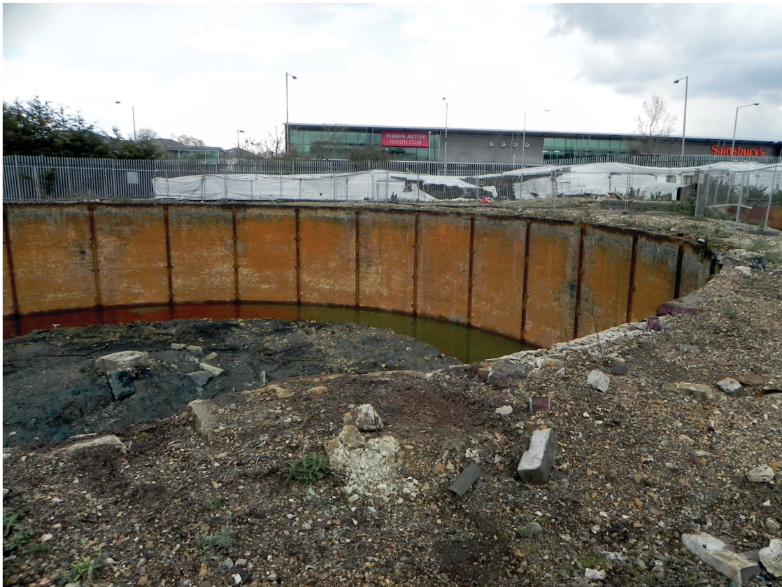
Fig 17 Gas holder 2 (see fig 1) outer wall, looking north
