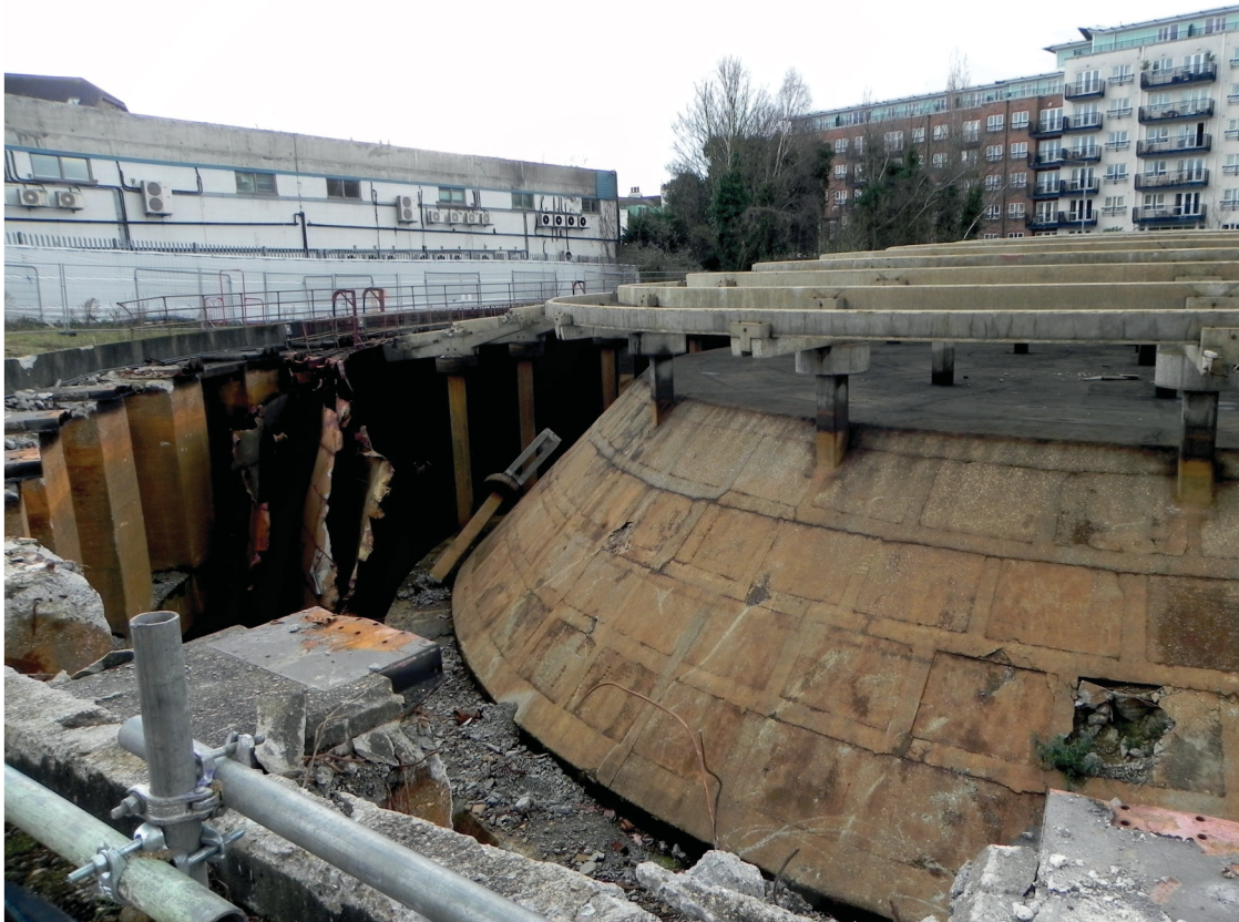
Fig 14 Gas holder 1 (see fig 1) substructure, looking south-west
