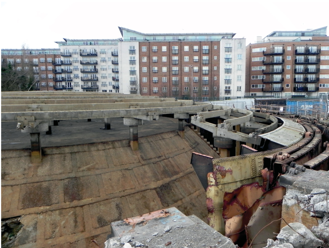
Fig 15 Gas holder 1 (see fig 1) substructure, looking north-west
