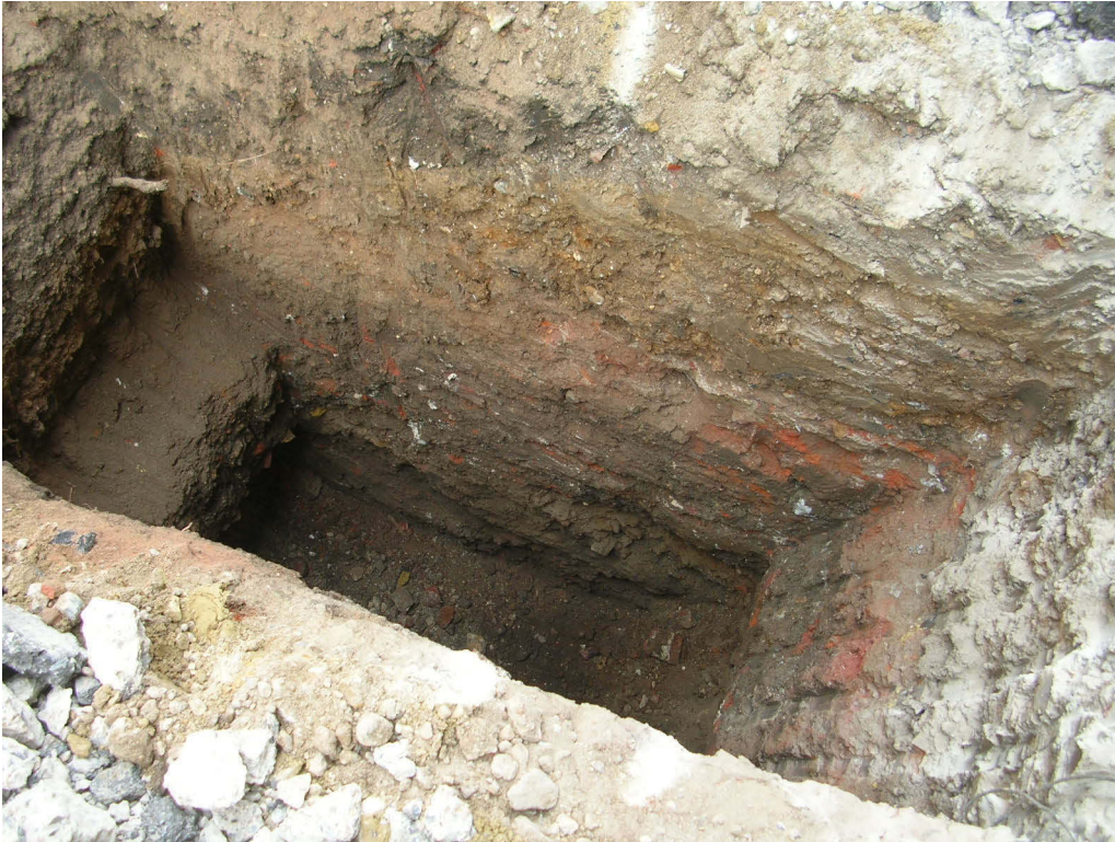
Trench E16 looking north
