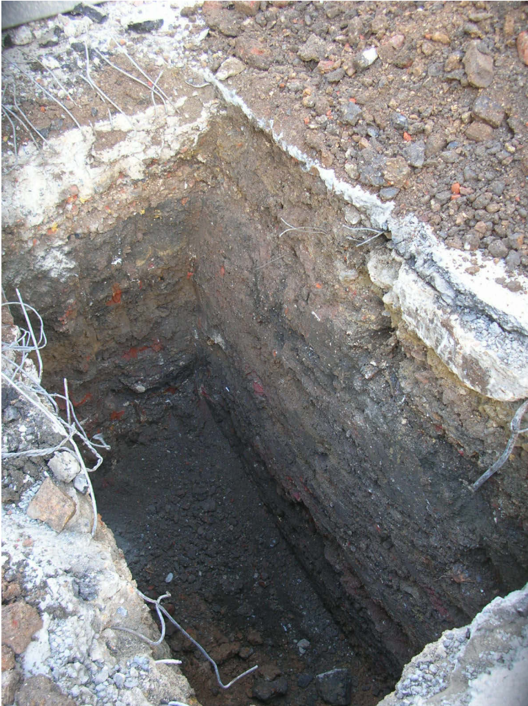
Trench E7 looking south west
