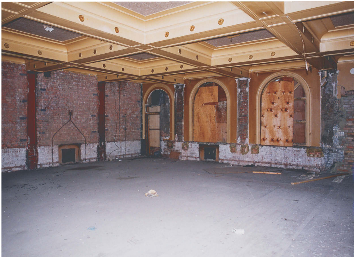
Fig 33 1F1, looking south-west (Tweeds 04/064)
