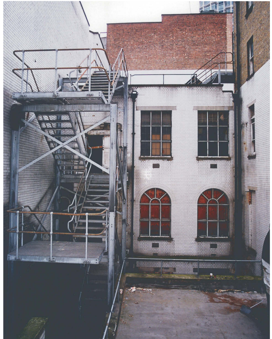
Fig 27 Exterior, rear north front, looking south (Tweeds 04/159)
