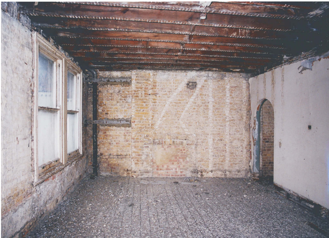
Fig 43 3F1/2, looking north (Tweeds 04/136)
