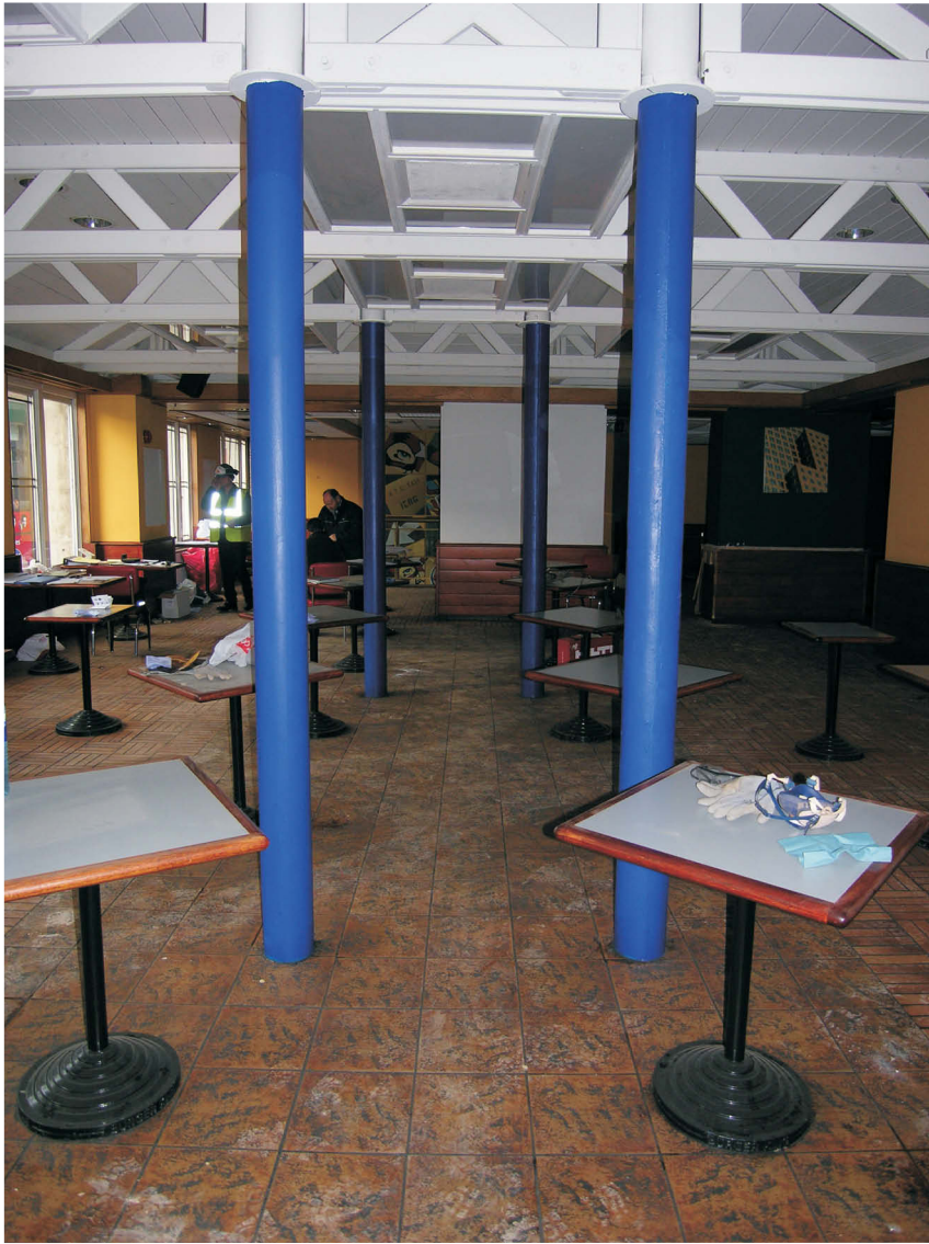
Fig 26 1F2, cast-iron columns, looking north (MoLAS 368//06/025)
