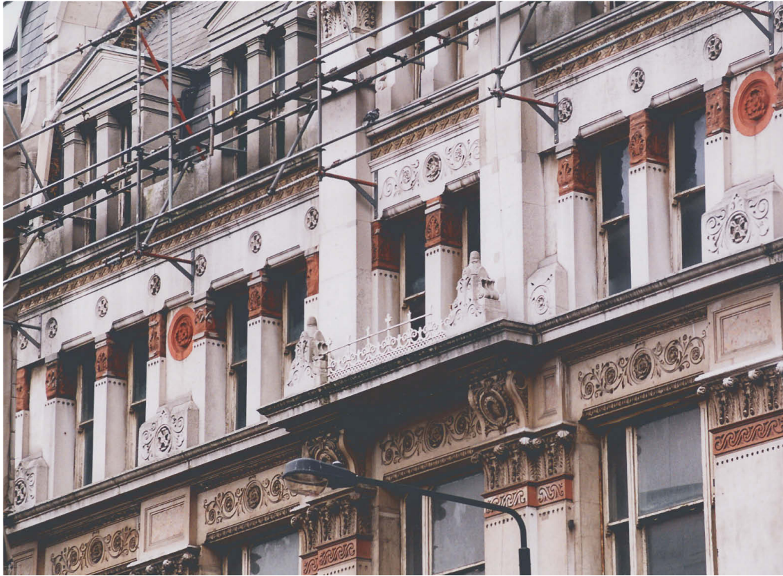
Fig 24 Exterior, west front, 2nd, 3rd and 4th floors (1875), looking north-east (Tweeds 04/123)
