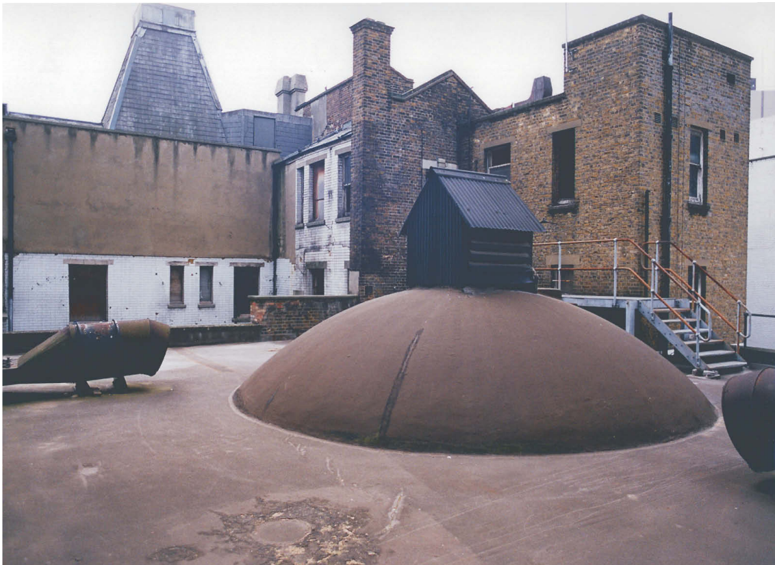
Fig 51 The roof of the Masonic Temple, looking west (Tweeds 04/073)
