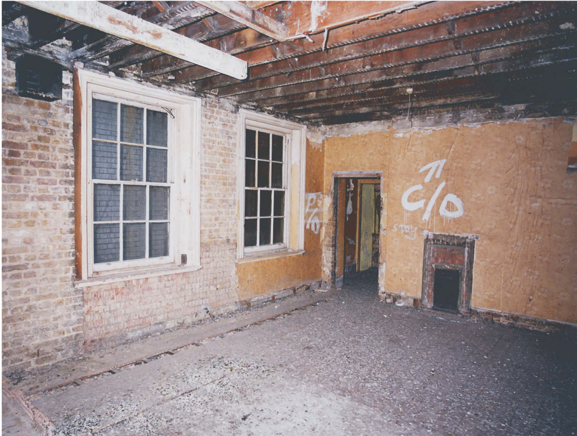
Fig 44 3F9/10, covered void for lift shaft in foreground. Looking south-east (Tweeds 04/142)
