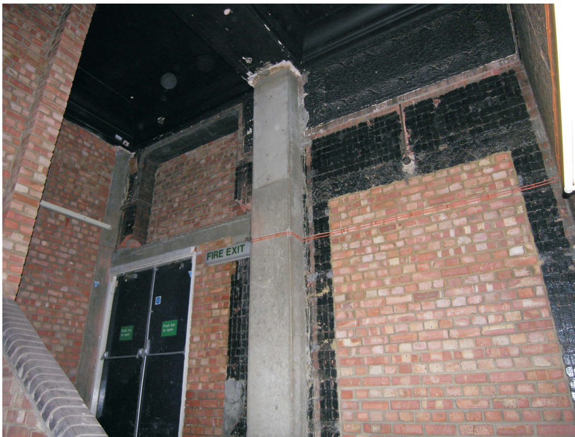
Fig 29 G1, blocked door and window openings, north wall, looking north (MoLAS 368/06/023)
