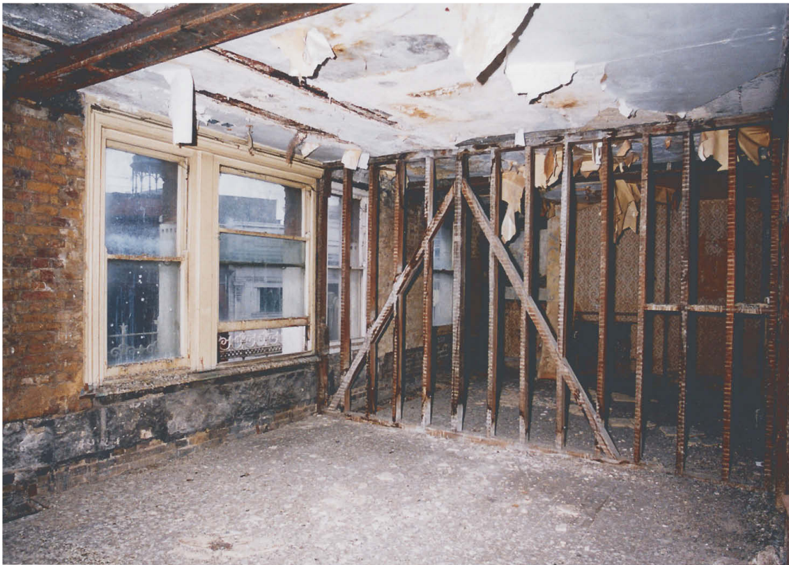
Fig 45 3F6/7, detail of timber frame and stud partition wall (Tweeds 04/037)
