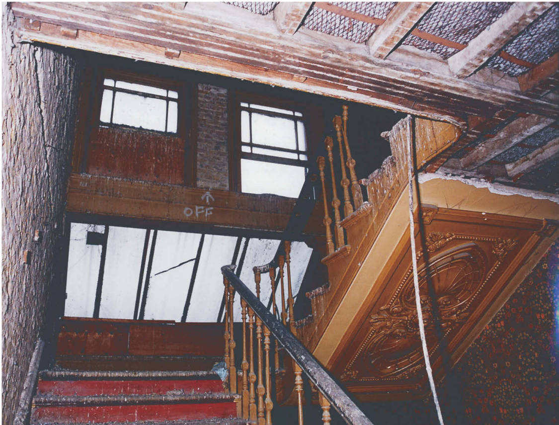
Fig 48 2F17, looking east from the 3rd floor (Tweeds 04/150)
