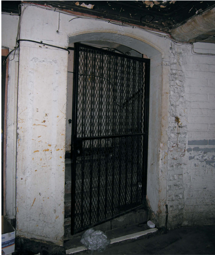
Fig 32 G2, arched opening and staircase in east wall, looking east (MoLAS 368/06/035)
