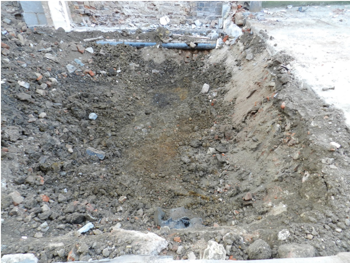
Gravel surface [7] looking north
