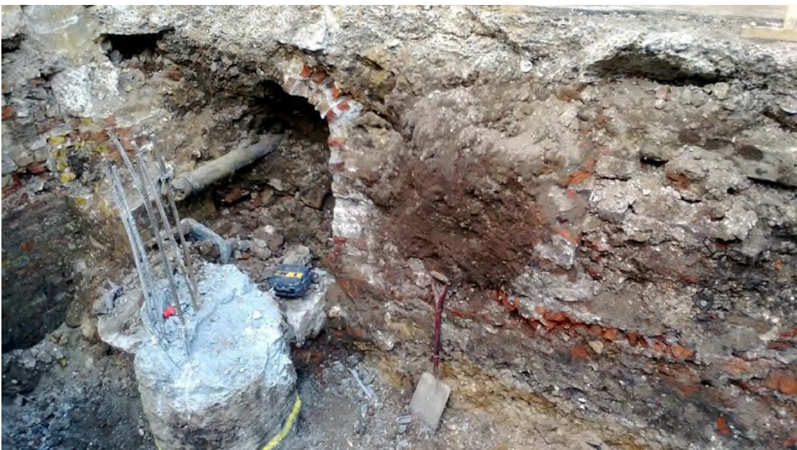
Fig 9 Photograph showing western end of south-facing section in trench along northern street frontage (secant pile trench 7), view to south
