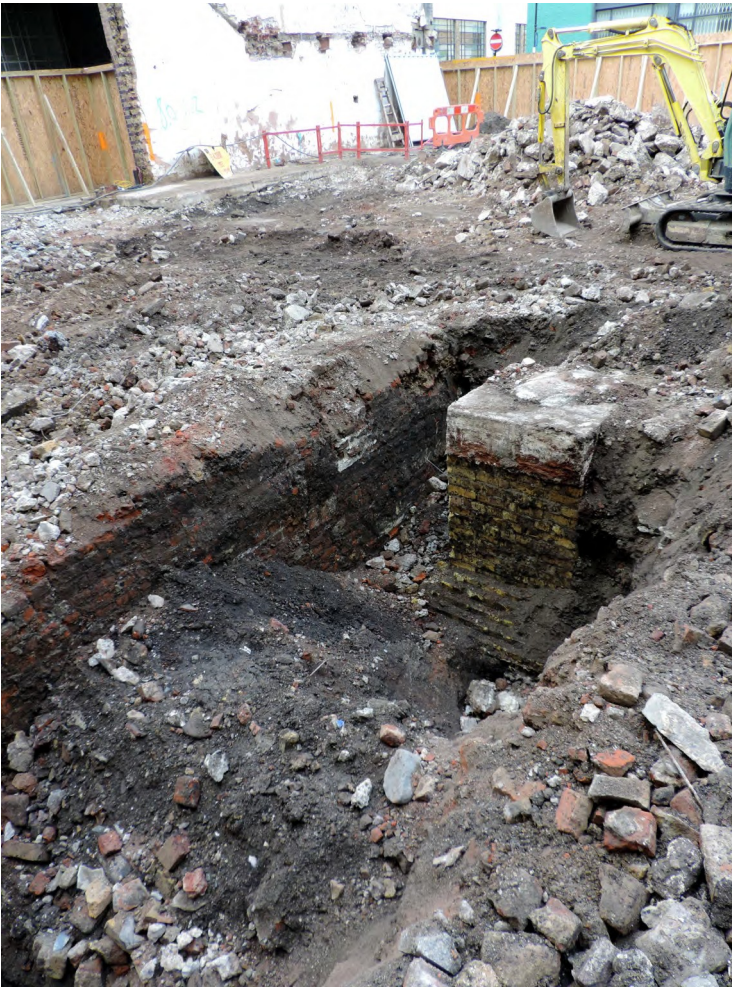
Fig 14 Brick wall running north-south across southern part of the site, view to north
