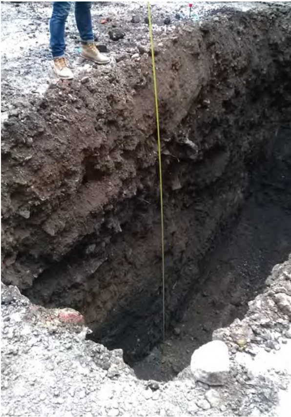
Fig 6 Photograph during machining of lift pit 1, view to northwest
