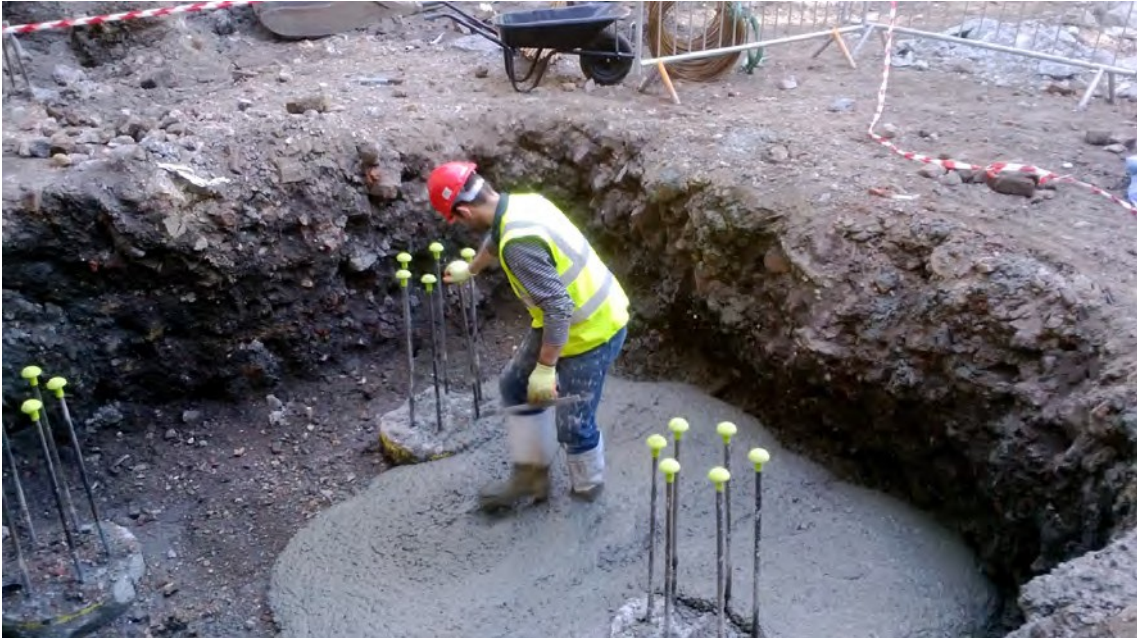
Fig 8 Photograph of east-facing section of pile cap 3, view to west
