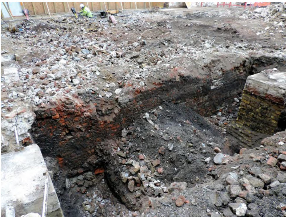
Fig 13 Brick wall running north-south across southern part of the site, view to northwest
