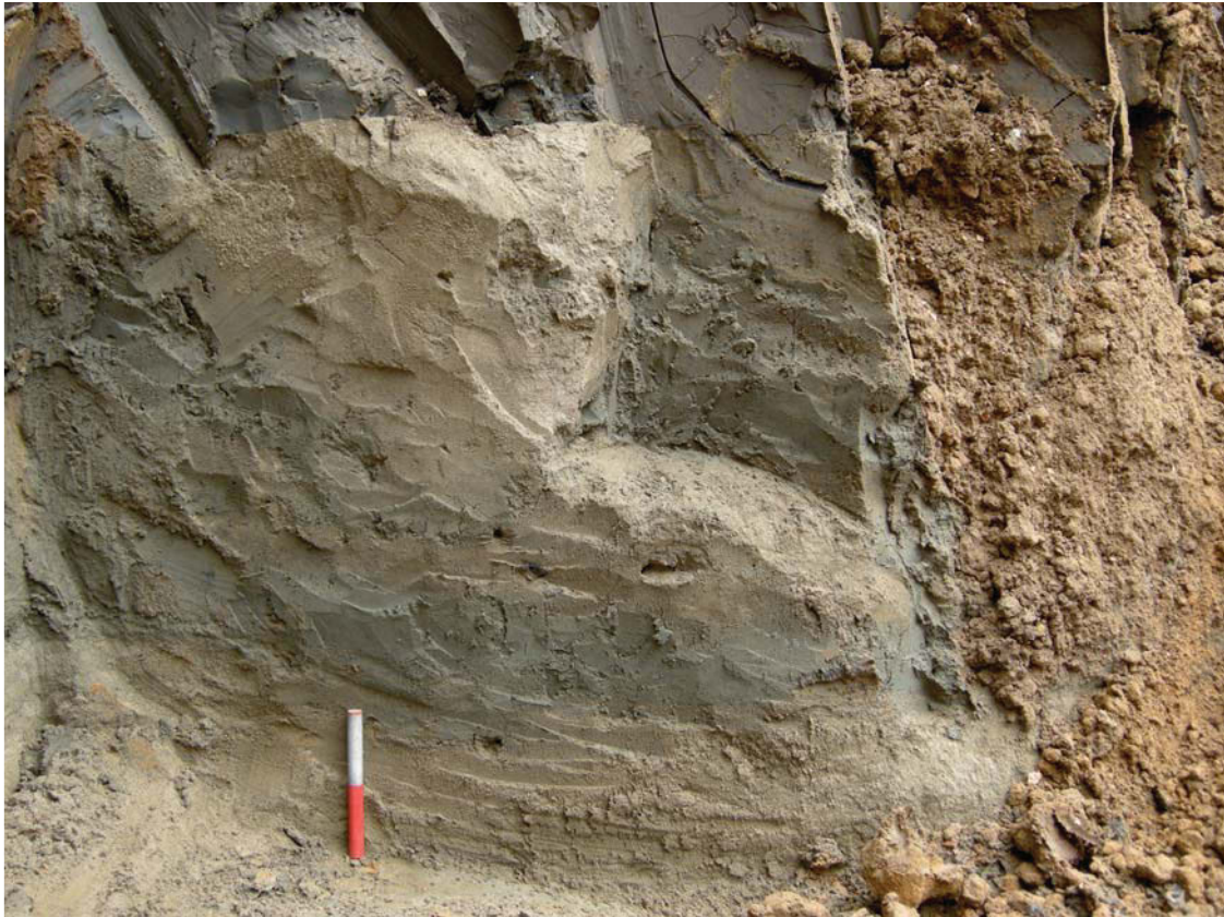
Fig 13 East area of channel [61] with lower fills [50], [60 and [63], looking north-east; 20cm scale
