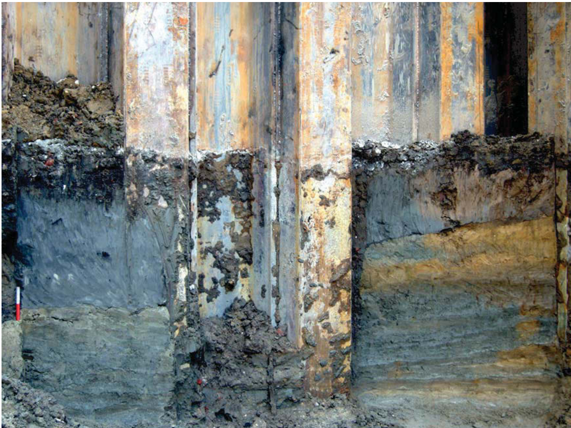
Fig 14 West area of channel [61] in section, looking south-west; a 20cm scale
