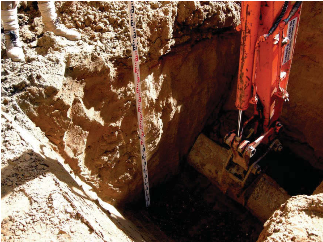
Fig 18 Exploratory slot through [67] exposing terrace gravels at base, looking south
