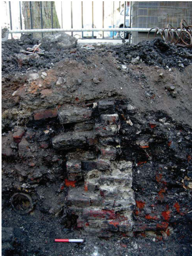
Fig 7 Wall [35], looking towards north-west; 20cm scale
